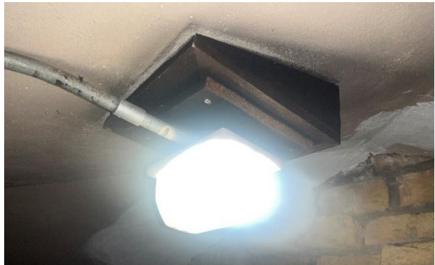
Figure 174. Surface-mounted non-original fluorescent light fixture at second-floor overlook level.
