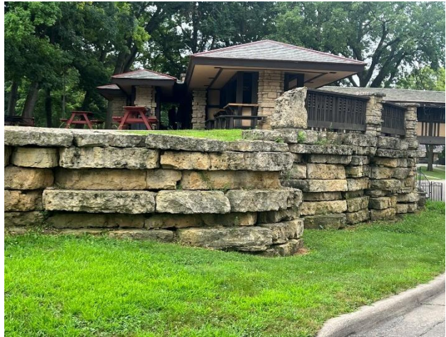
Figure 54. Dry-laid stone retaining, as viewed from the north.
