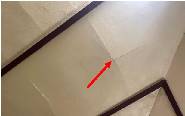
Figure 202. Irregular cracking pattern where sagging was observed.
