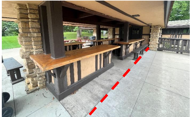
Figure 376. Concrete floors at the covered patio and north terrace. Note that the concrete at the covered patio is different than the concrete at the north terrace.
