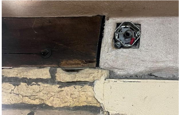
Figure 280. Historic junction box that supported a light fixture adjacent to the door at the south room.
