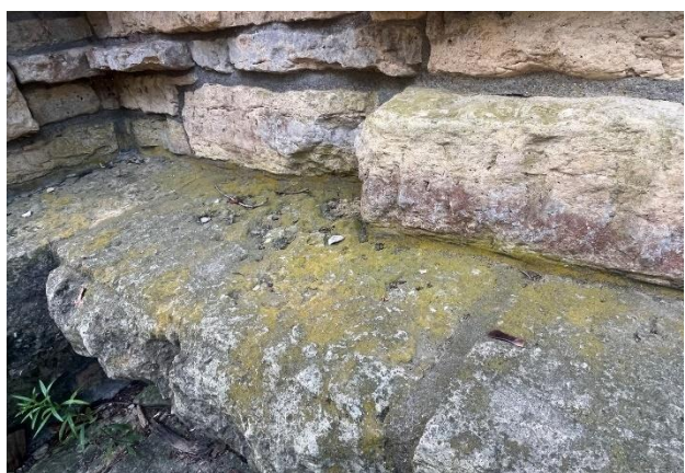
Figure 300. Biological growth and soiling at upward-facing surface.
