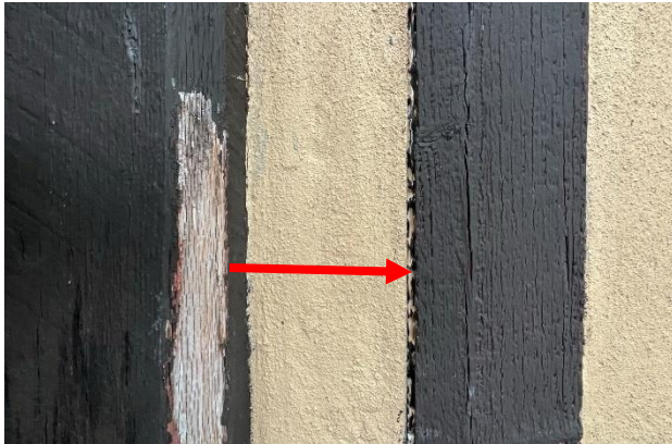
Figure 509. Gap between stucco wall framing and wood post framing.
