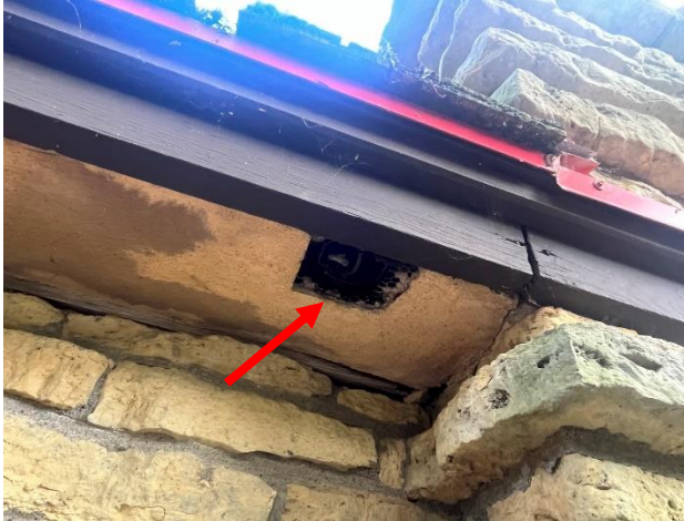
Figure 332. 7-inch square opening in stucco eave.
