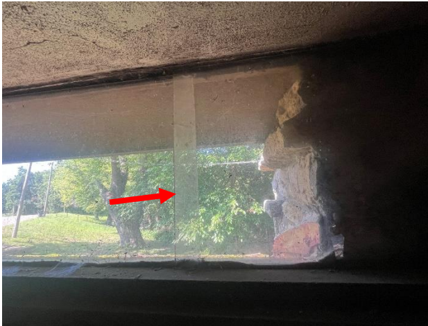
Figure 335. Dormer window with overlapping acrylic panel glazing and no dividing mullion.
