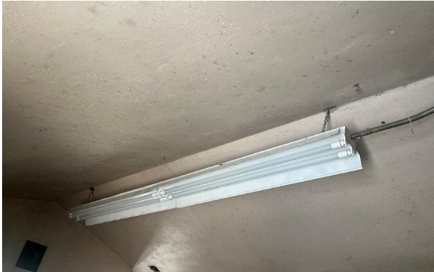
Figure 289. Non-original double ballast fluorescent light fixture suspended along the interior ridge of the roof.
