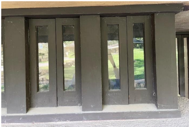
Figure 248. Close up view of wood casement windows.
