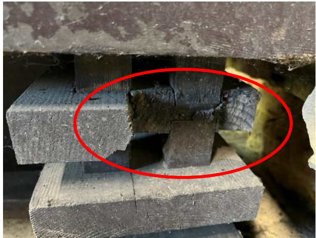
Figure 199. Missing portions of the decorative 2x8 wood members are missing.
