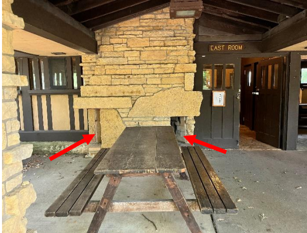
Figure 418. Two exterior fireboxes, one at each corner.
