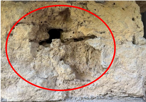
Figure 299. Stone unit with deep pockets and pits.
