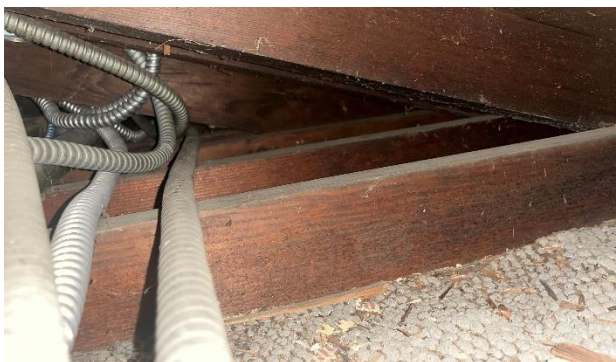
Figure 435. Conduit extending through open eave framing in roof.
