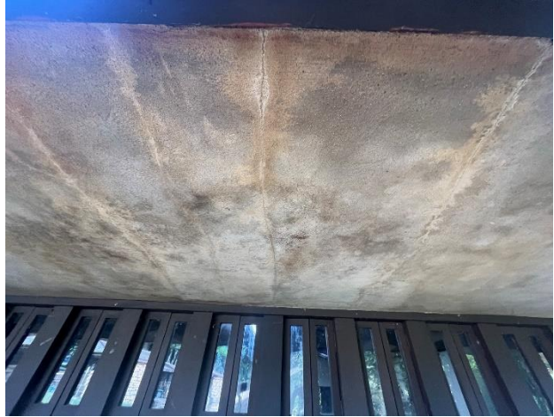
Figure 329. Cracks spaced approximately 14 inches apart with discoloration around the crack.
