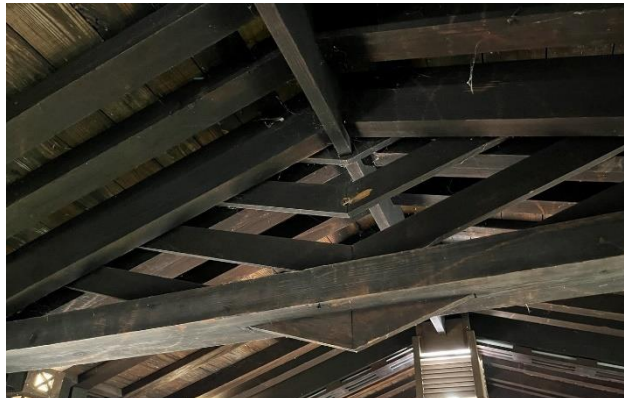
Figure 327. Roof framing with chevron pattern wood slats at bridge roof.
