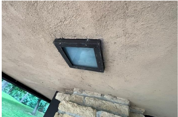
Figure 357. Recessed light fixtures in the soffit.
