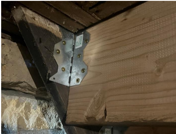
Figure 144. Non-original 2x10 riser secured to the stringer with stainless steel angles.
