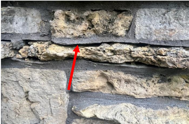
Figure 450. Spalling and erosion of stone along a mortar joint.
