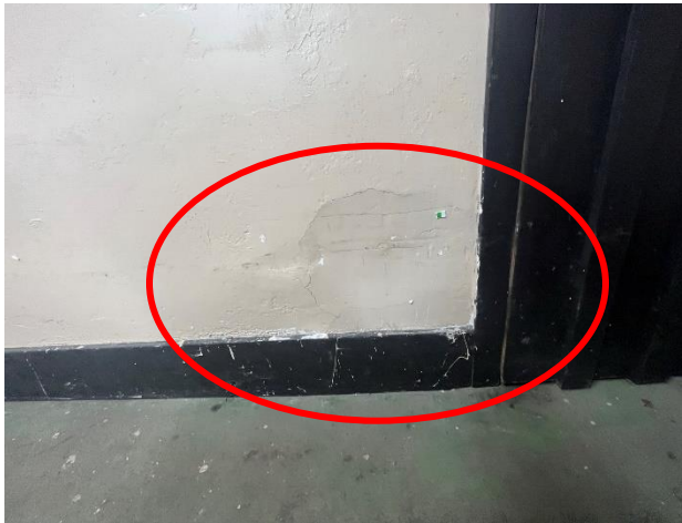
Figure 323. Localized area of damaged plaster at the wall separating the north and south rooms.
