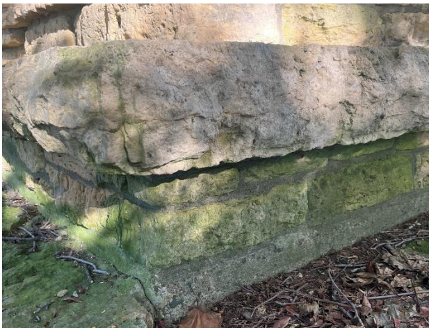
Figure 301. Biological growth and soiling around the base of the building.
