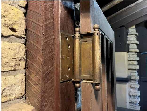
Figure 415. Original double-action hinge at door.
