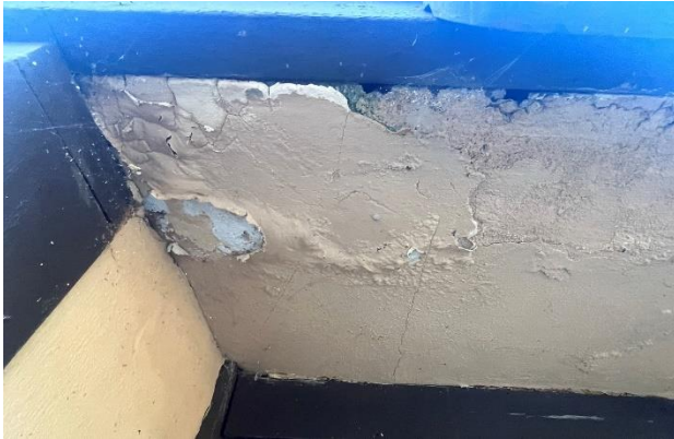
Figure 334. Peeling paint at the stucco soffit.
