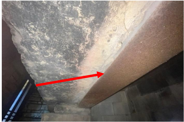
Figure 185. Surface corrosion at the steel angle that supports the mantel.
