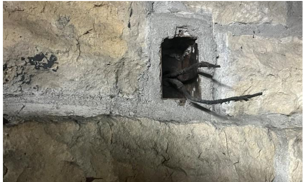
Figure 284. Abandoned switch in storage closet with cloth-jacketed wiring.
