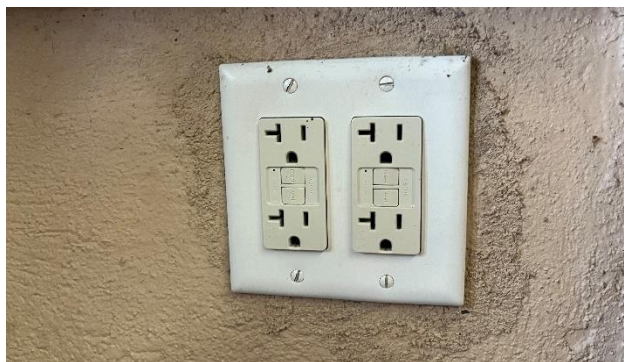
Figure 436. Non-original GFCI receptacle set into wall. Note evidence of previous plaster repair around the outlet.
