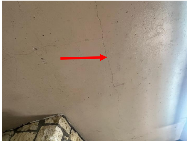
Figure 326. Hairline cracking extending perpendicular to each other and over the full length of the room.
