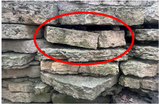
Figure 453. Cracking extending the full depth of the stone, with stone displaced.
