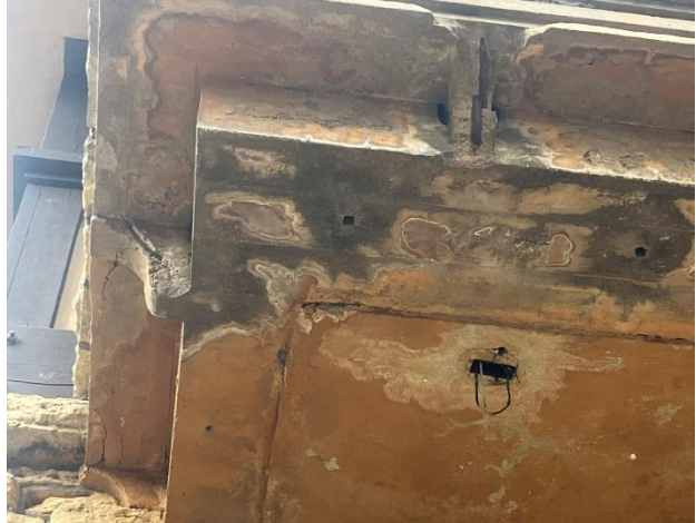
Figure 488. Moisture staining at the concrete at the underside of the balcony.
