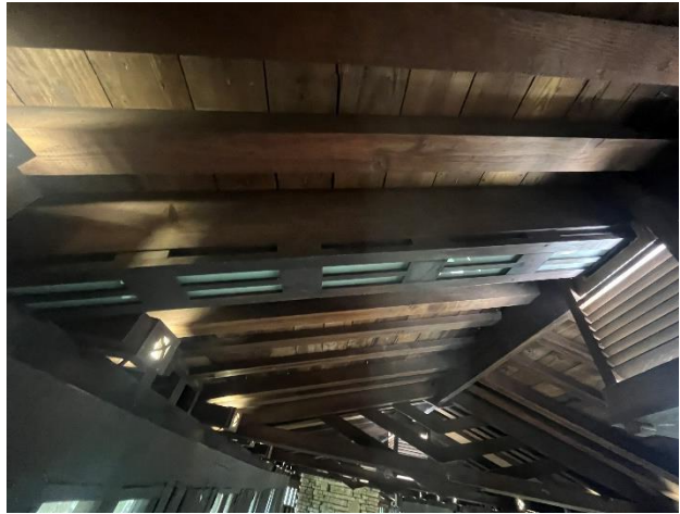
Figure 440. Wood panel, adjacent to lantern-style light, mounted to roof rafters to create a light box.
