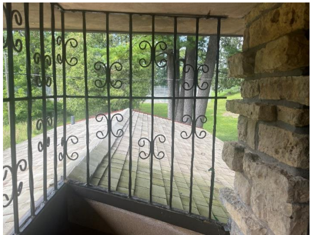
Figure 120. Non-original wrought iron rail mounted to the wood balustrade rail and to the underside of the stucco soffit.
