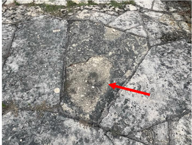
Figure 455. Surface spalling at the face of a stone unit.
