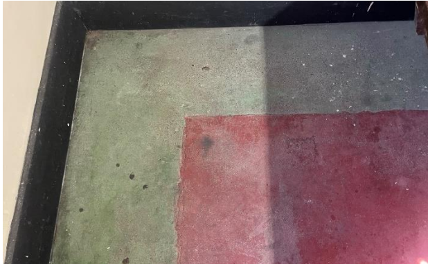
Figure 264. Thin cementitious floor topping, measuring 3/16 inch thick, that has colored aggregate and has been painted.
