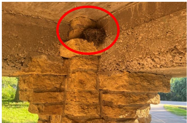
Figure 504. Bird's nest at recess between stone units.
