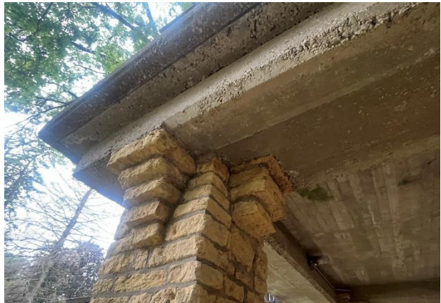
Figure 367. Edge of the concrete deck slab.
