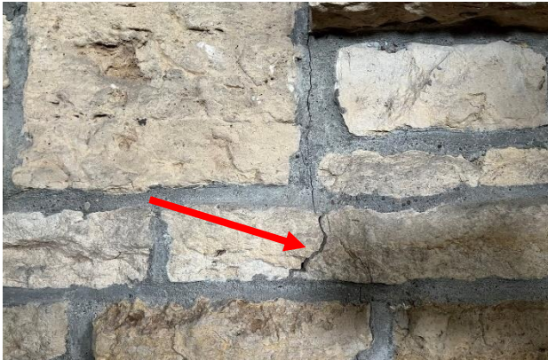
Figure 464. Vertical cracking at west room fireplace.
