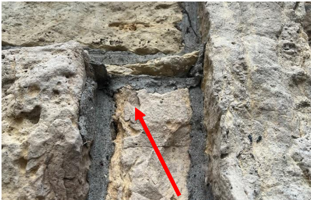
Figure 478. Chipped stone ledge unit.
