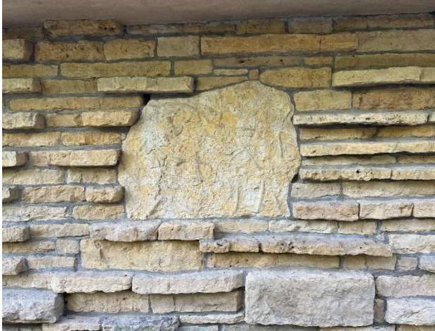
Figure 241. The face bed stone unit.
