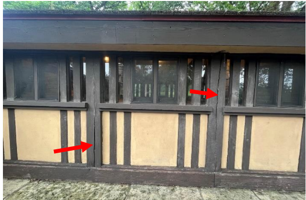
Figure 492. Vertical splits in wood post framing, viewed from exterior.
