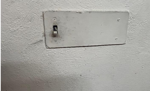
Figure 283. Original light switch in south room with non-original blank-off panel reducing the panel to a single switch.
