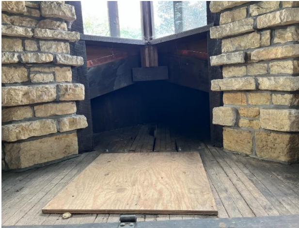
Figure 409. Wood tongue-and-groove flooring at lookout tower.
