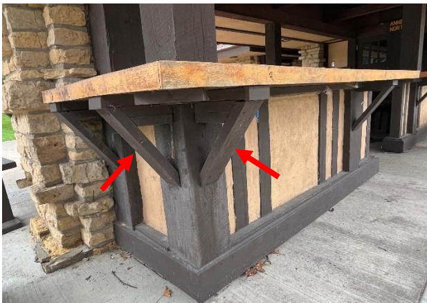
Figure 379. View of 2x wood members supporting the wood counter above.
