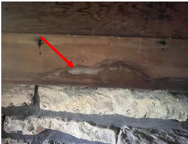
Figure 221. Moisture staining and white-colored soiling along the bottom framing member.
