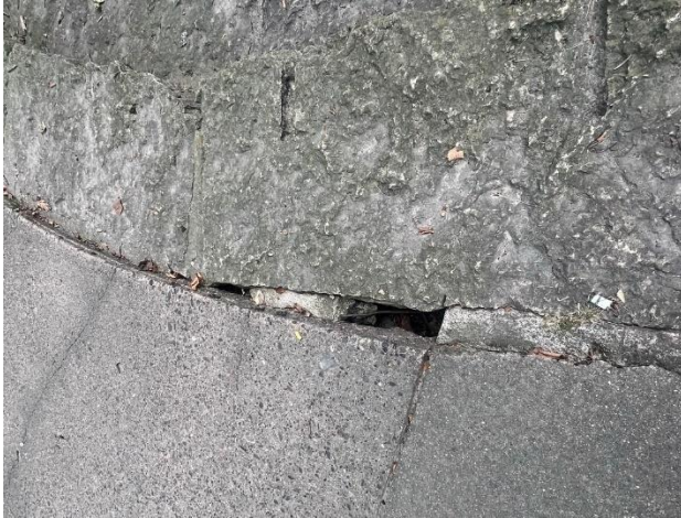
Figure 487. Open joint between concrete sidewalk and stone stair.
