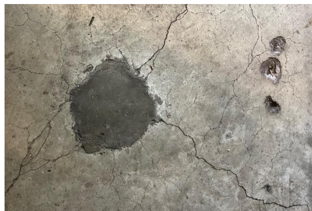
Figure 485. Cracking and spalling at the concrete flooring of the north annex.
