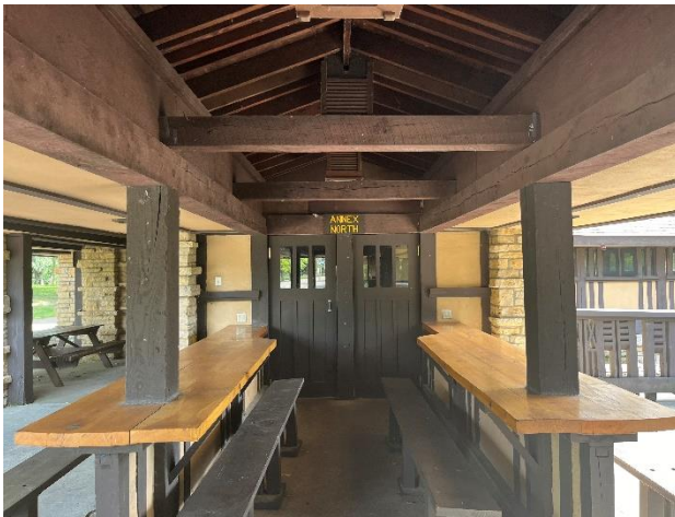
Figure 377. Exposed roof framing at the center of the space and stucco clad soffits at the edge of the space.
