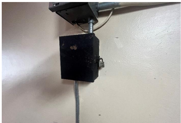
Figure 288. Sub-panel surface-mounted to wall at north room.
