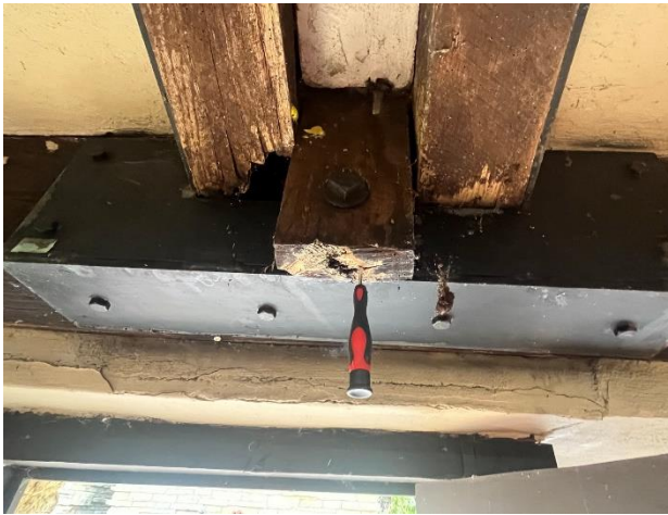
Figure 308. Awl probing soft and rotted wood.
