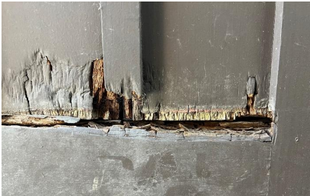
Figure 337. Distress at bottom end of door panels.
