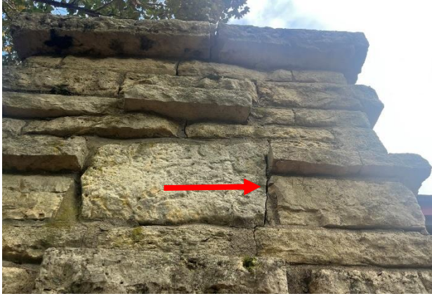
Figure 291. Vertical cracking at the exterior west elevation of the north chimney.
