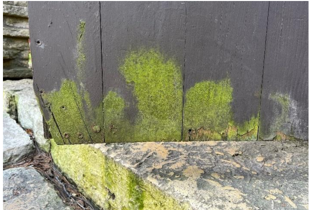
Figure 216. Minor wood deterioration at doors including biological growth.
