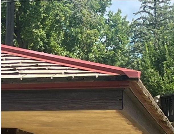
Figure 112. An aluminum drip edge wrapping around the wood fascia.
