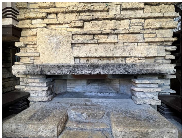
Figure 147. Stone mantel spanning across the firebox opening.
