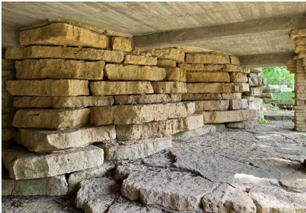
Figure 366. Dry-laid stone retaining wall within the covered stone terrace.
