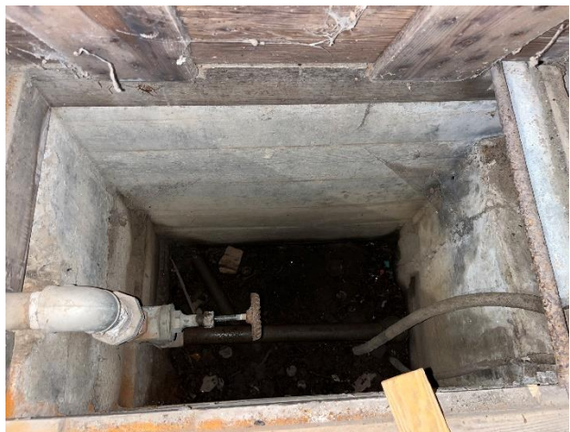
Figure 177. Concrete pit concealed under wood flooring that provides access to main water supply.
