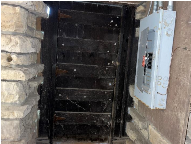
Figure 141. Horizontal reinforcing on the mechanical room face of the door.
