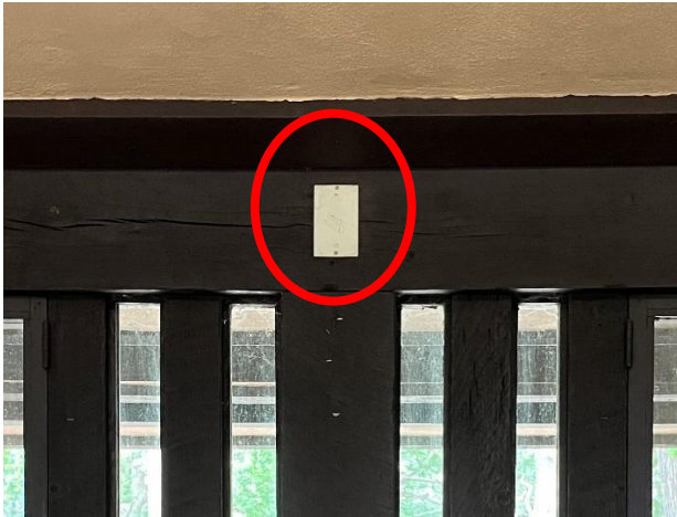
Figure 449. Cover plate over abandoned junction box.
