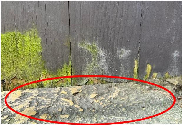
Figure 215. Isolated areas of peeling paint.
