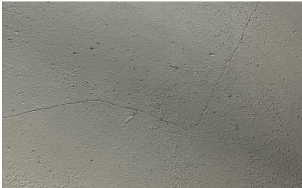
Figure 204. Incrementally stepped cracking across the plaster surface.
