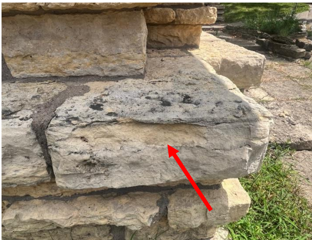
Figure 186. Shallow spalls at edge of stone units.
