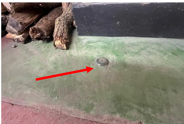
Figure 268. Cap from previously existing radiator system.
