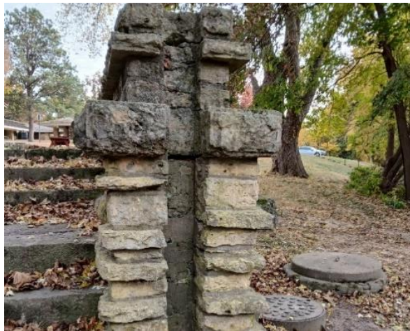
Figure 38. Channel cut into stone walls at Veranda Rooms.
