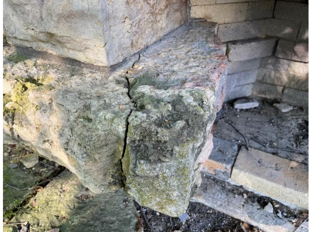
Figure 320. Cracked stone unit adjacent to steel lintel.
