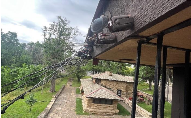
Figure 431. Main utility line attached to wood fascia at west elevation of building.
