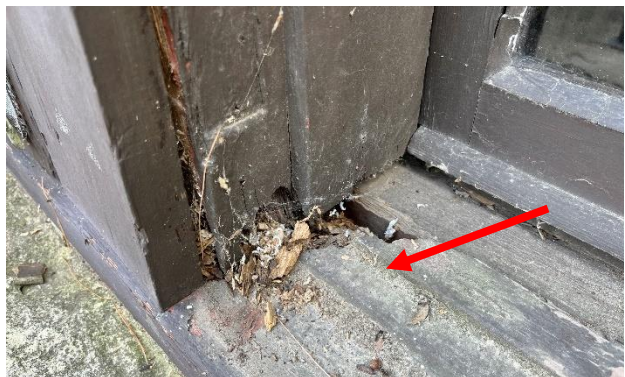
Figure 214. Localized area of wood that was found to be soft when probed, with small splits and checks at the end of framing members.
