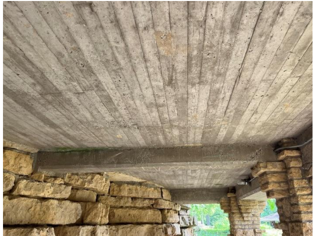
Figure 365. Concrete deck with slab with formboards.
