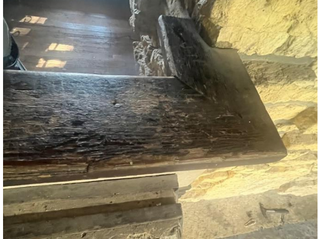
Figure 129. The top of the balcony walls have a wood 2x8 top rail.
