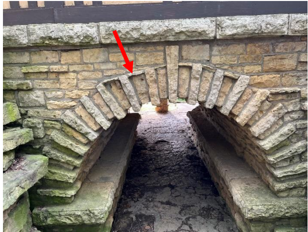
Figure 371. Stone voussoir at the stone archway with the stone drip edge units indicated by arrow..
