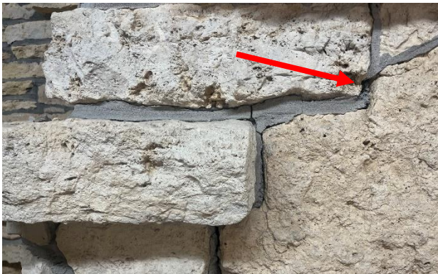
Figure 293. Open mortar joint at cracked stone unit.
