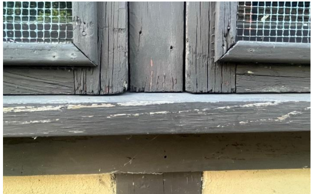
Figure 338. Distress at the top surface of a window sill.
