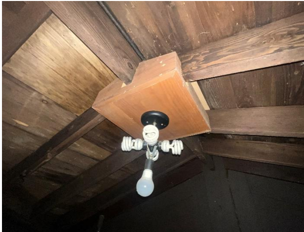
Figure 445. Non-original wood light fixture mounted to roof framing at the east room.
