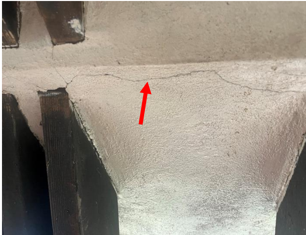
Figure 325. Hairline crack extending perpendicular between roof rafters.
