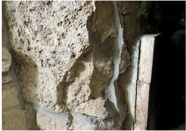
Figure 469. Spalled stone unit adjacent to firebox.
