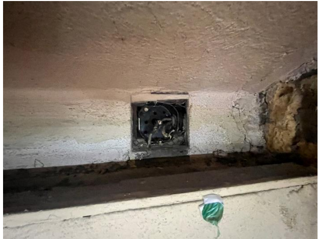
Figure 278. Cloth-jacketed electrical wire within the junction box.
