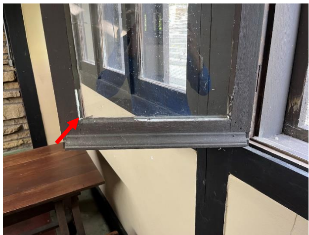
Figure 340. Casement window with deteriorated glazing putty.
