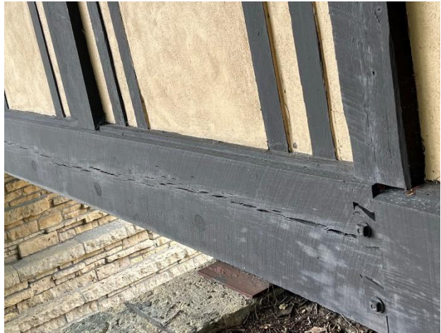
Figure 496. An approximately 20-foot-long split extending through the middle of the wood beam at the east portion of the south bridge framing member.
