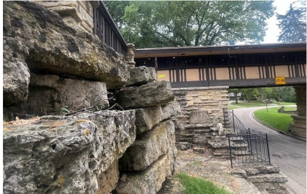
Figure 63. Displacement of stone units and bulging of the wall was most prevalent approximately 6 feet above grade.
