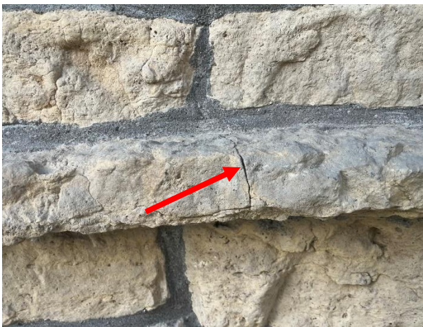
Figure 295. Crack running vertically through the stone.
