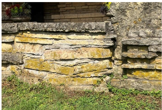
Figure 65. The stone paving and parapet wall adjacent to the coping unit are displaced and partially collapsed.
