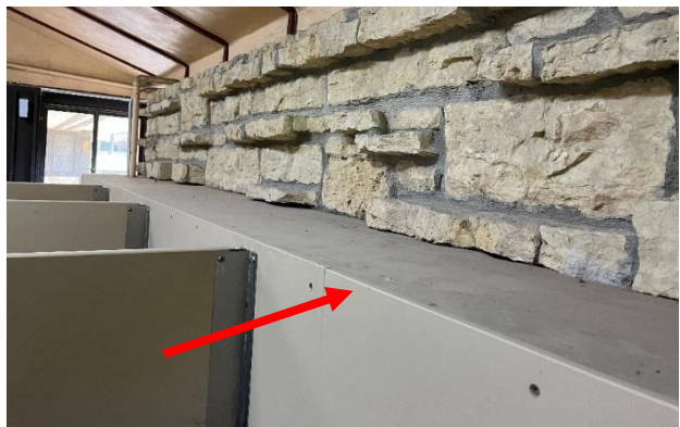
Figure 131. Gypsum board finish (arrow) concealing the plumbing pipes and conduit for the toilets and sinks.
