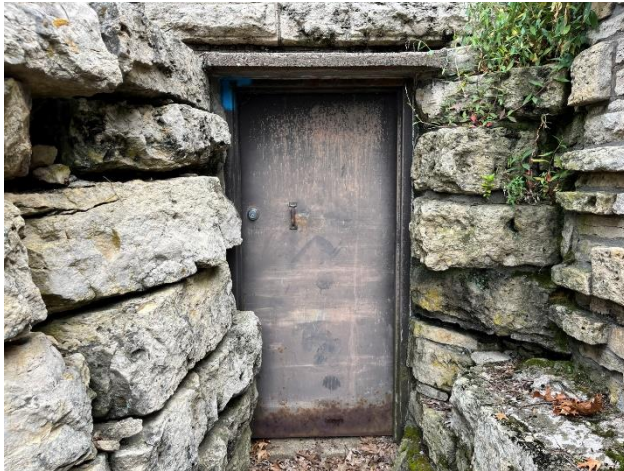
Figure 349. Non-original steel-framed door.
