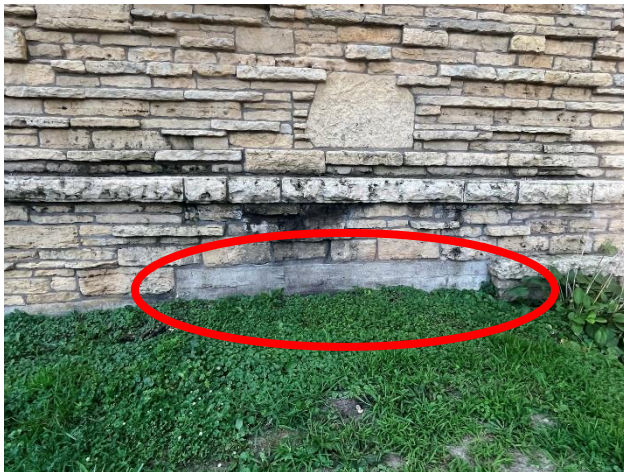
Figure 316. Cast-in-place curb above foundation visible on the south elevation of the west reservoir.
