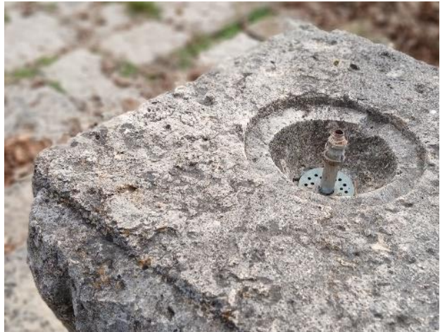
Figure 46. Bubbler pipe in stone next to amphitheater.
