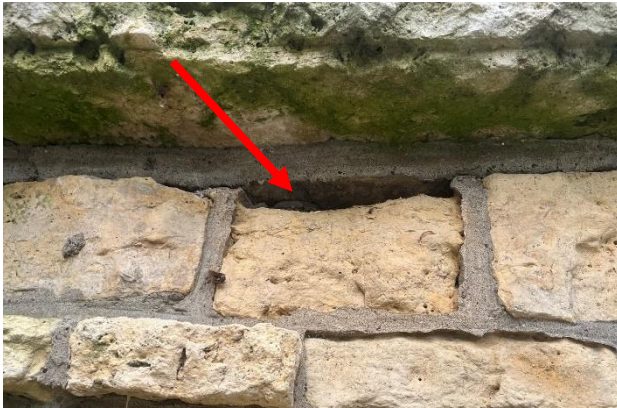
Figure 452. Spalling and erosion of stone along a mortar joint.
