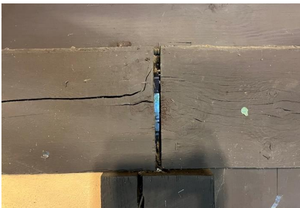
Figure 493. Separations at joint between wood framing members.
