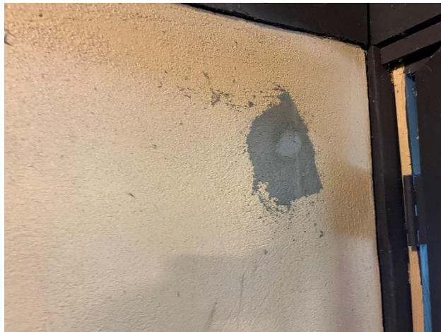
Figure 512. Unpainted patch at previous patch repair.
