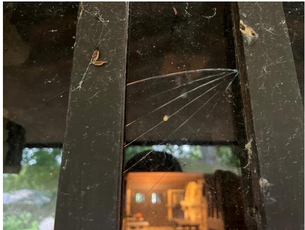
Figure 519. Cracked glass light at door.
