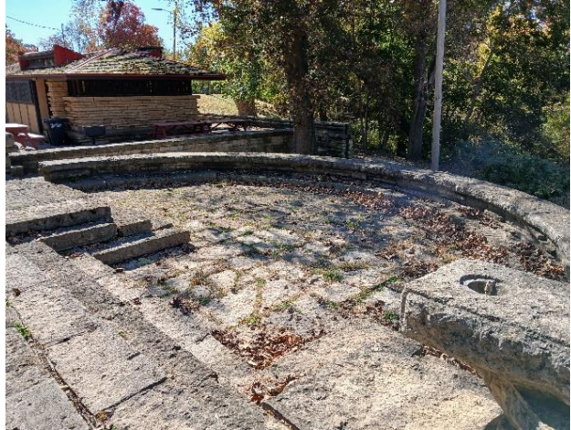
Figure 44. Circular wall and steps of amphitheater. Note irregular blocks of limestone pavement.
