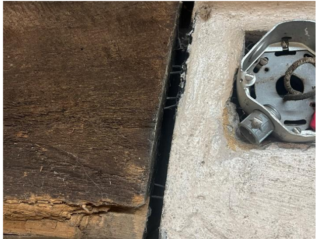
Figure 313. Joint, 1/2 inch wide with visible nails.
