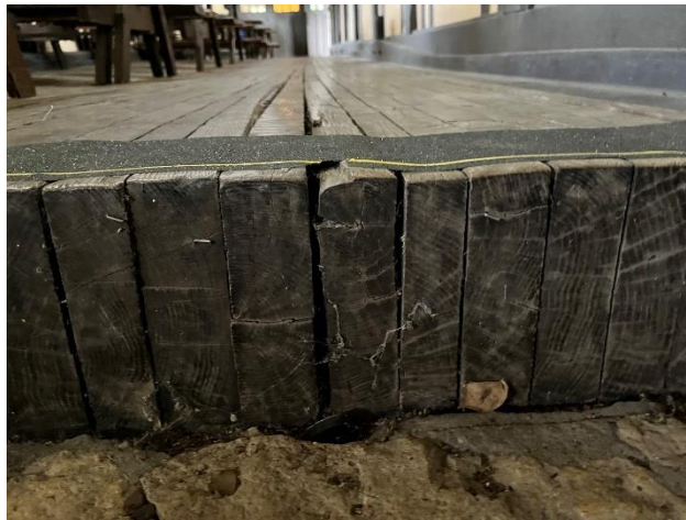
Figure 402. Ends of wood deck framing members.
