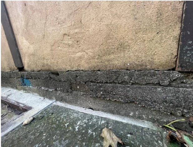
Figure 229. Exposed concrete foundation and floor slab exposed on east elevation.
