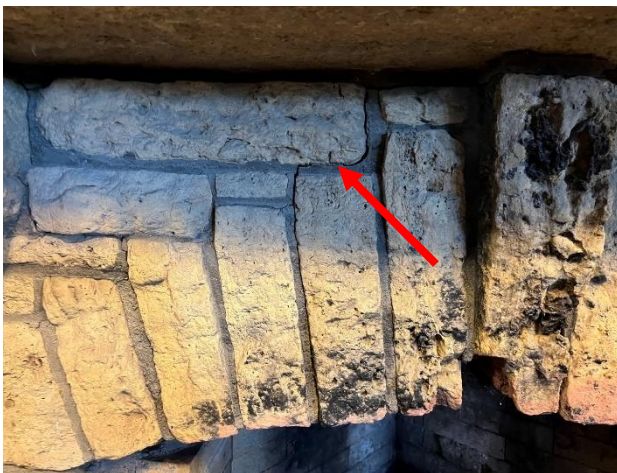
Figure 466. Cracking at stone below mantel at east room fireplace.
