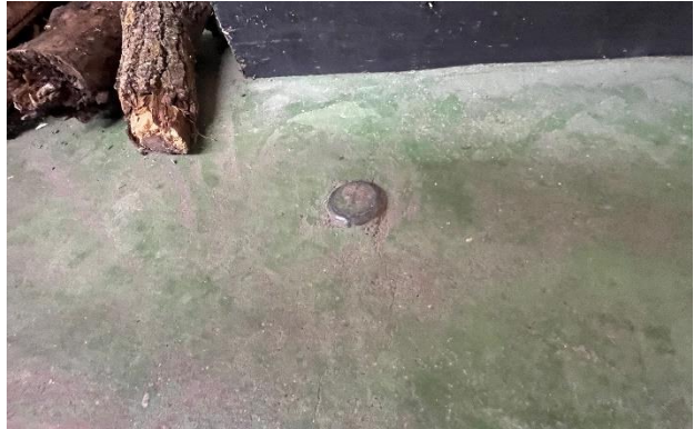
Figure 290. Cap of pipe where radiant heating unit was located.
