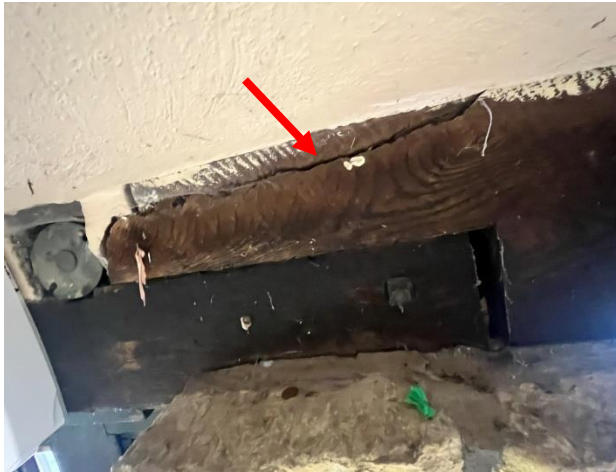
Figure 312. Indication that the south beam may be sagging.
