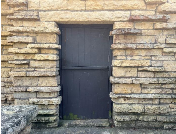
Figure 98. Dutch door with a stone lintel.
