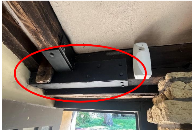
Figure 236. Structural repairs made to the beam and rafters at the north end of the east dormer.
