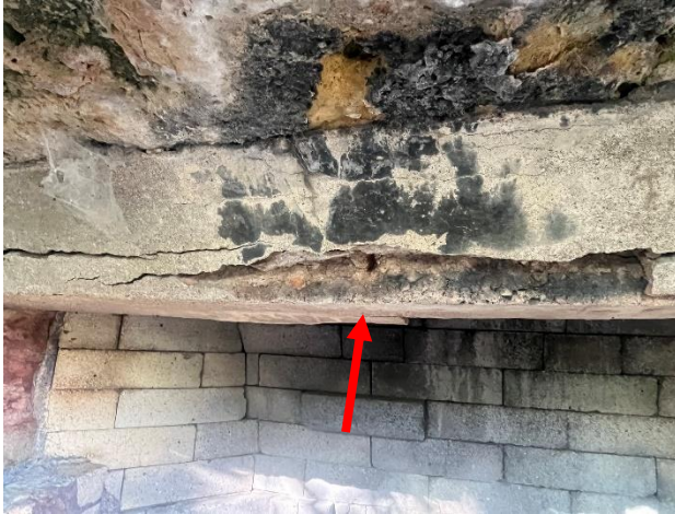
Figure 319. Spalls at concrete lintel aligning with steel reinforcing.
