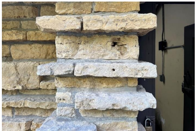
Figure 238. Typical stone units and coursing at building corners.
