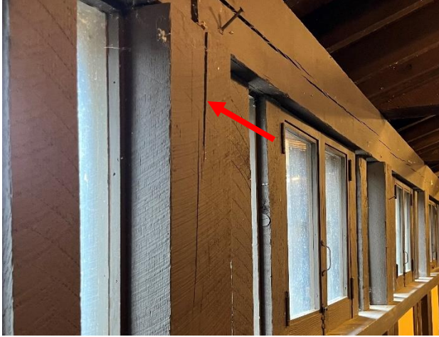
Figure 489. Vertical split in wood post framing viewed from interior.
