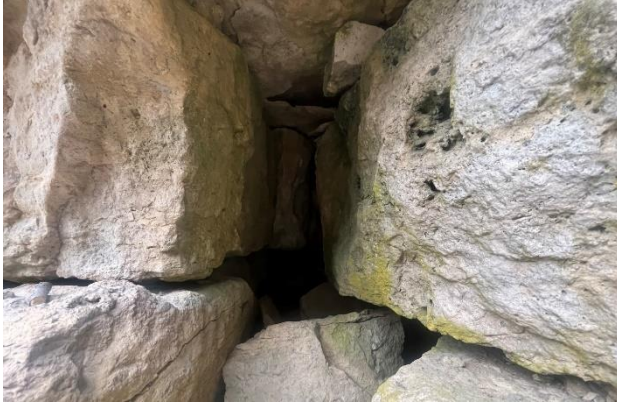
Figure 60. Large voids were observed at the joints between stone units at the retaining wall that extends under the north terrace and south end of the east pavilion.
