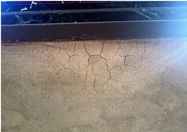
Figure 330. Map cracking along the edge of the eave.
