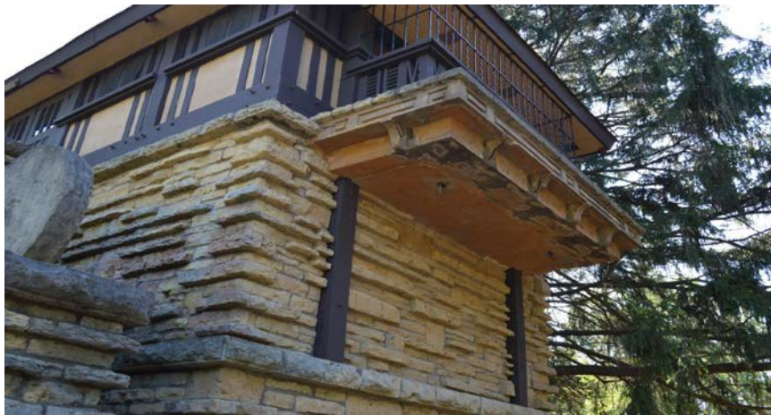
FIGURE 8 Detail of the western end of the Bridge Complex, showing the deterioration of the balcony and its missing lighting fixtures. Source: Photograph by Dr. Julie Schlarman September 14, 2015.
