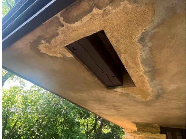
Figure 333. Previous stucco patch.
