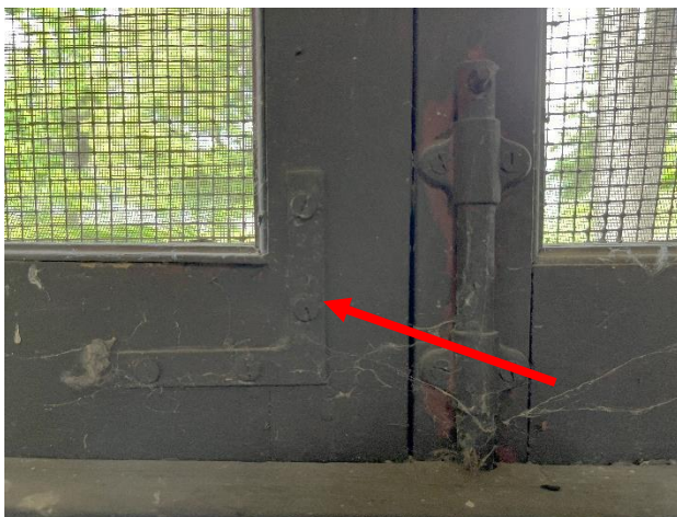
Figure 219. A previous repair that includes the addition of metal brackets to reinforce the sash corners.
