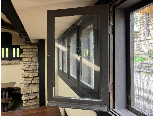
Figure 253. Casement sash at east window bay.
