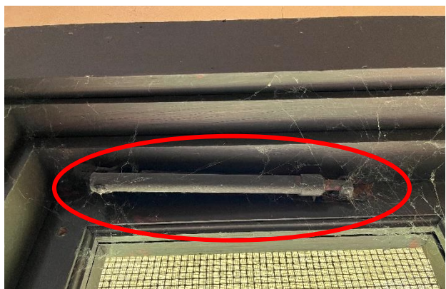
Figure 90. Typical hardware includes a hydraulic hinge at the top of each window sash.
