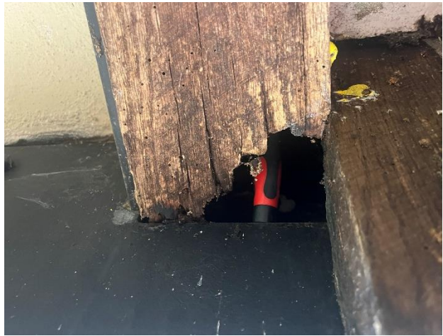
Figure 309. Wood framing exhibiting over a 50 percent section loss.
