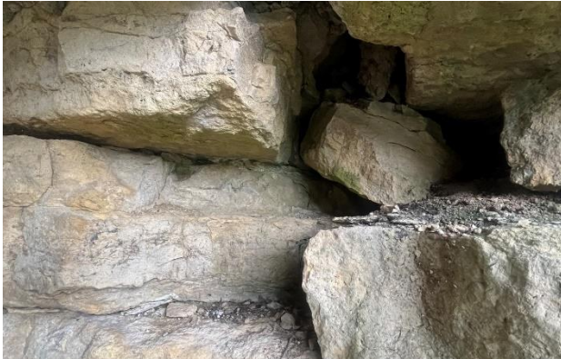
Figure 62. The voids measured as much as 6 inches wide and to a depth of a few feet.
