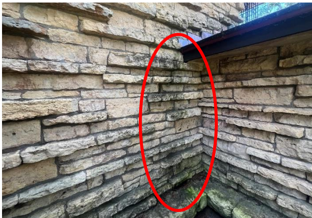
Figure 192. Biological growth and soiling at stone walls perpendicular and adjacent to roof runoff.
