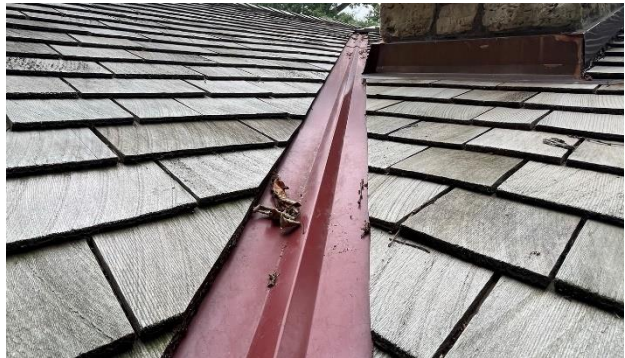
Figure 351. Valley flashings with triangular break.
