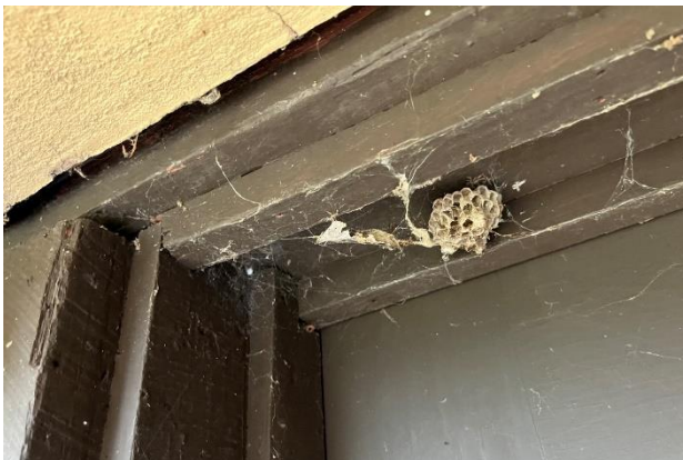
Figure 503. Insect nest at wood window framing.
