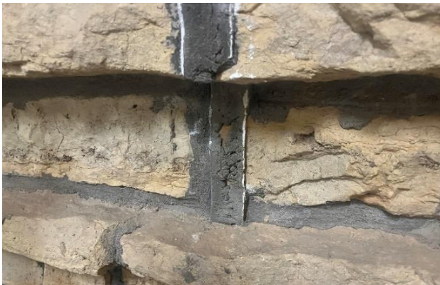
Figure 132. Evidence of previously existing interior partition wall.
