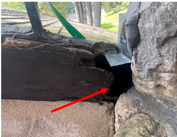
Figure 194. Complete section loss at the wood top rail and trim at the exterior balconies.
