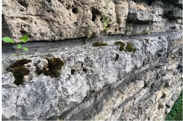
Figure 475. Plants and biological growth at the stone cladding.
