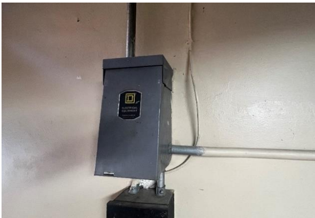
Figure 287. Surface-mounted electrical panel in the north veranda room. Note the black sub-panel below.
