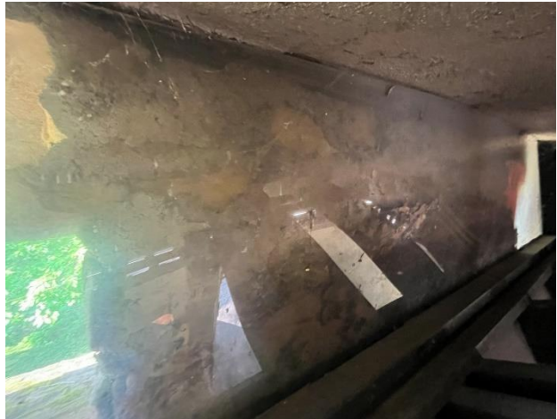
Figure 336. Bowing due to built-up debris between dormer window and chimney.
