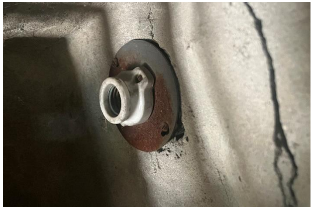
Figure 282. Historic light fixture with a circular metal plate and porcelain light socket.
