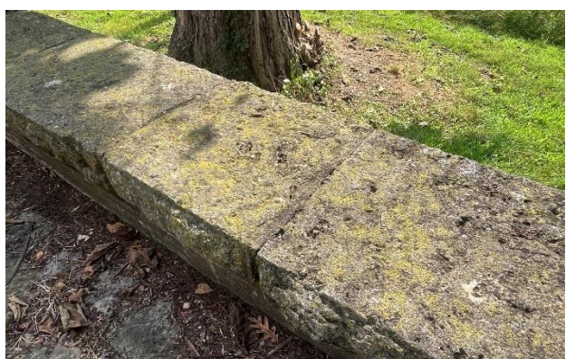
Figure 71. Moss and lichen were observed at most of the stone parapet walls.
