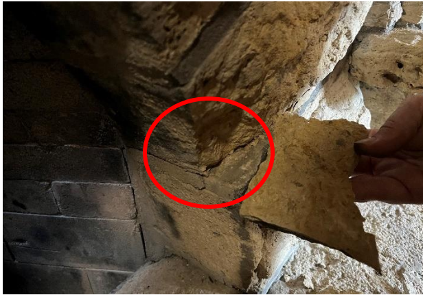
Figure 188. Shallow spalls at the stone unit around upper fireplace opening.
