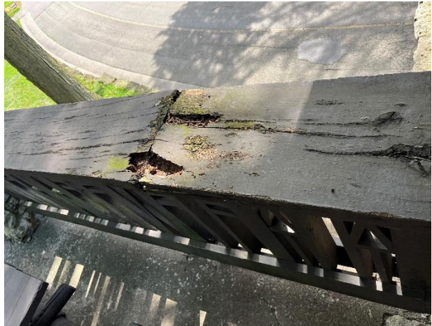
Figure 500. Severe deterioration and biological growth at wood of top rail of railing.
