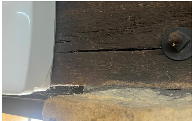
Figure 311. Checking at the ends of a beam aligned with anchor locations.
