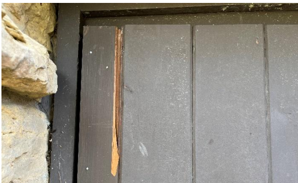
Figure 213. Split at upper leaf of Dutch door.
