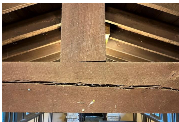
Figure 494. Split along the center of a roof beam that spans across the east room.
