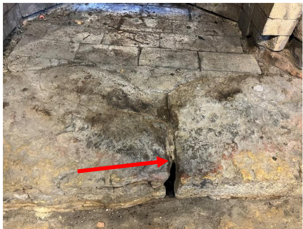
Figure 467. Open joint at hearth stone.
