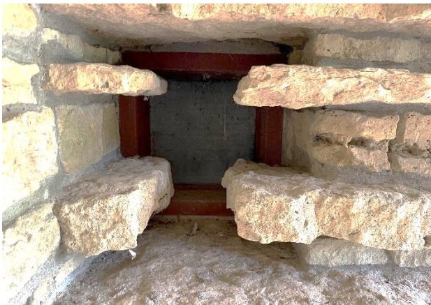
Figure 95. Wood-framed casements that are operable from the interior.
