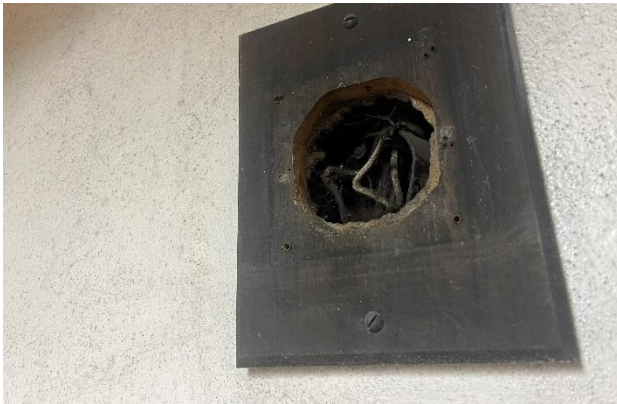
Figure 279. Evidence of historic light fixture and wood back plate.
