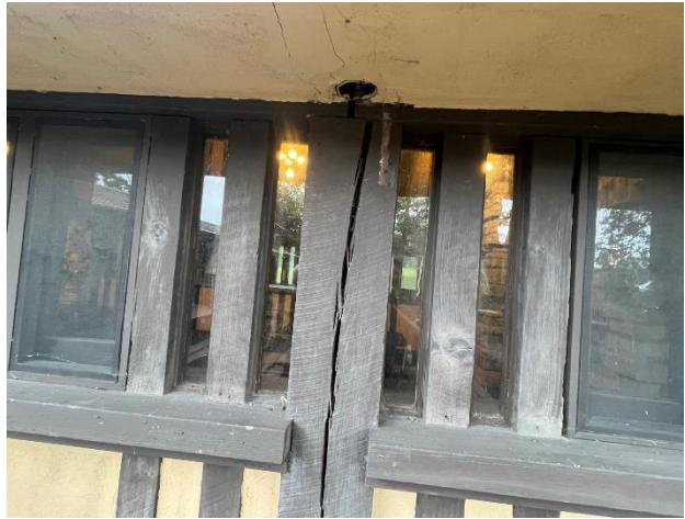
Figure 490. Vertical split in wood post framing, viewed from exterior.
