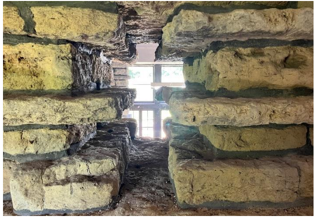
Figure 149. Irregular-shaped opening in the chimney.
