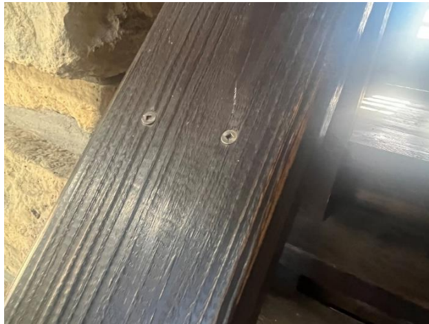
Figure 145. Top rail consisting of a 2x6 secured to the posts with screws.
