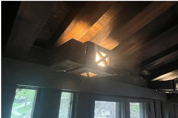
Figure 441. Wall sconce at interior of bridge is set between roof rafters.
