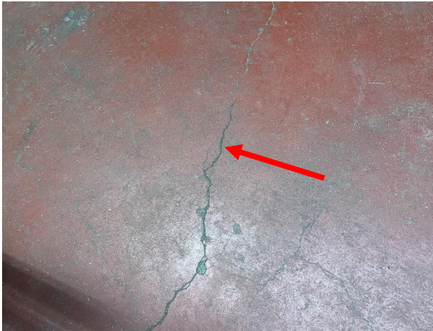
Figure 306. Cracking at interior floor of north Veranda Room.
