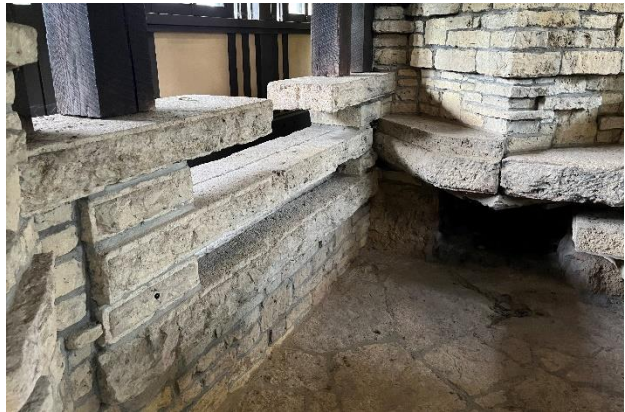
Figure 427. North knee wall, consisting of alternating long and short stone units.
