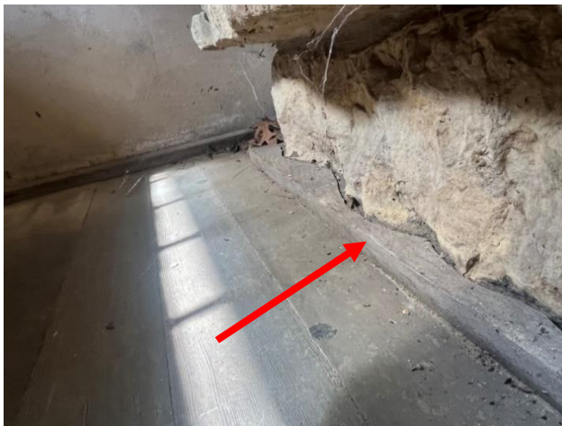
Figure 121. Rounded base trim board notched around the stone.
