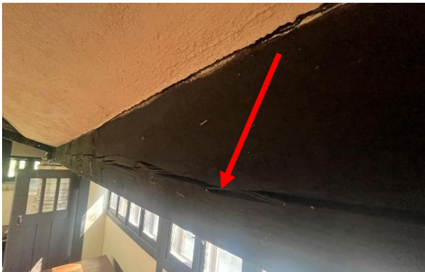
Figure 310. Large area of checking at mid-height of wood beam.
