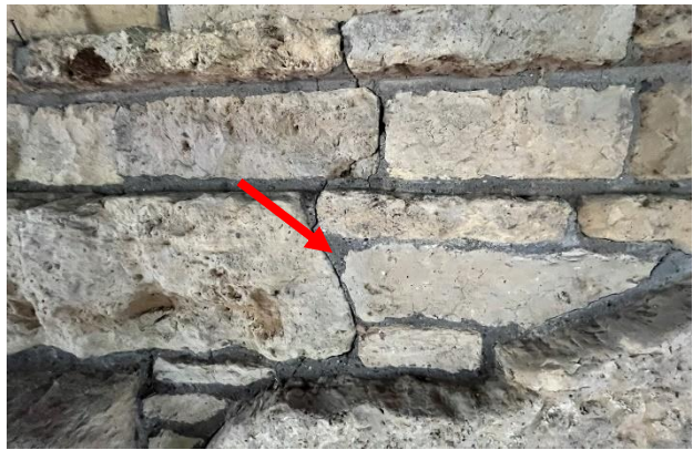
Figure 463. Vertical cracking at west room fireplace.
