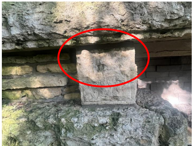
Figure 318. Spalled stone unit below corroded steel plate.
