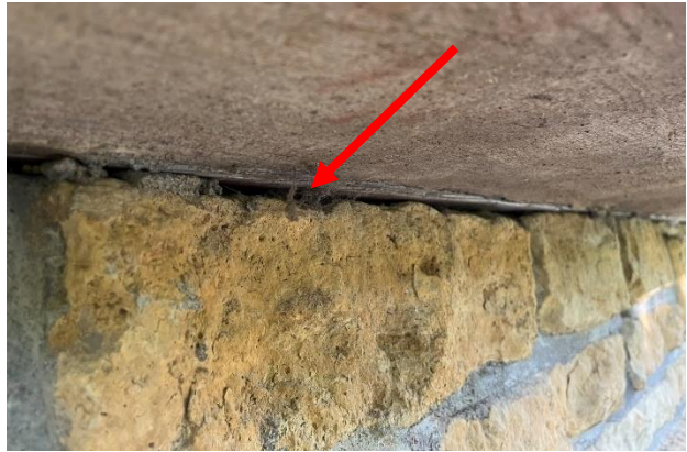
Figure 298. Open joint at the interface between the stucco eave and stone wall.
