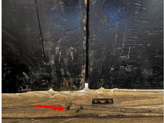
Figure 109. A hole in the flooring that appears to have been for a receiver for a surface-mounted floor latch.
