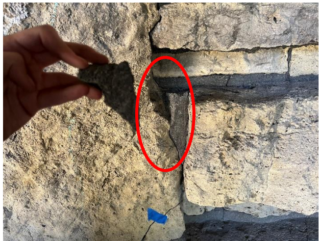
Figure 187. Small spall at face bed unit above the lower fireplace mantel.
