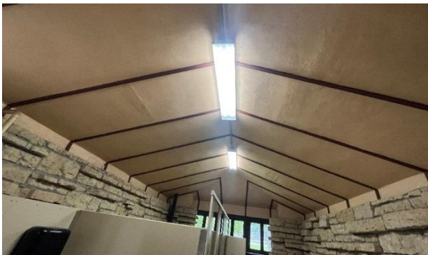
Figure 175. Non-original double ballast box-shade fluorescent light fixtures at the men's and women's restrooms.
