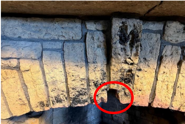
Figure 470. Spall at the bottom of the stone keystone at the fireplace mantel.
