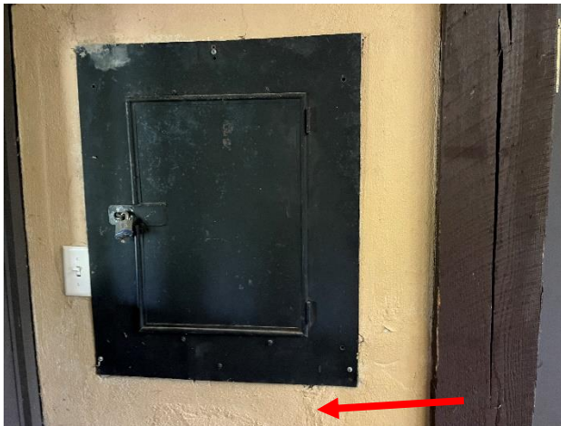
Figure 511. Vertical hairline crack extending from the corner of a non-original electrical box.
