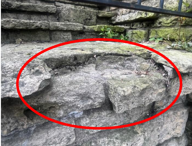
Figure 456. Localized spall the full depth of a stone paver.
