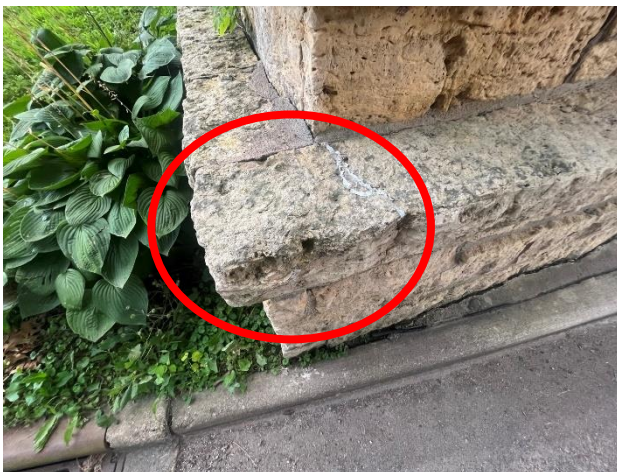
Figure 472. Previously repaired crack. The stone unit was unsound when tapped with a mallet.
