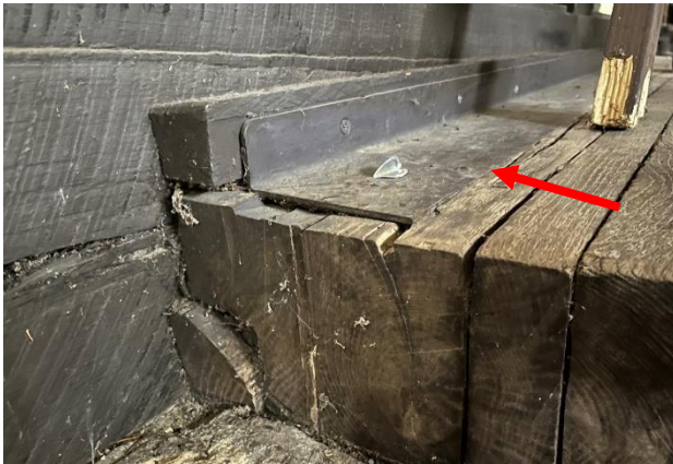
Figure 405. Edge of wood deck bridge framing showing steel angle.
