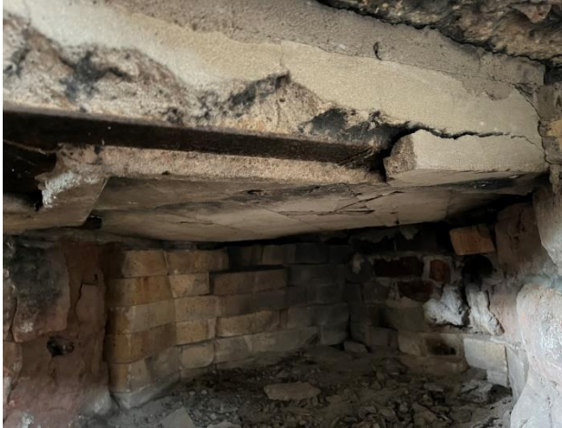
Figure 481. Spalled concrete exposing the metal lintel over the west fireplace.
