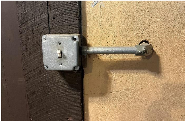
Figure 437. Non-original surface-mounted conduit and light switch.
