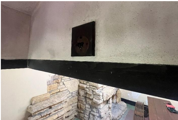
Figure 281. Junction box that historically supported a light fixture at the south window cove.
