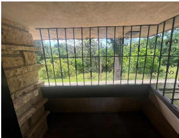
Figure 119. Second-floor exterior balcony with partial-height stucco-clad balustrade walls.
