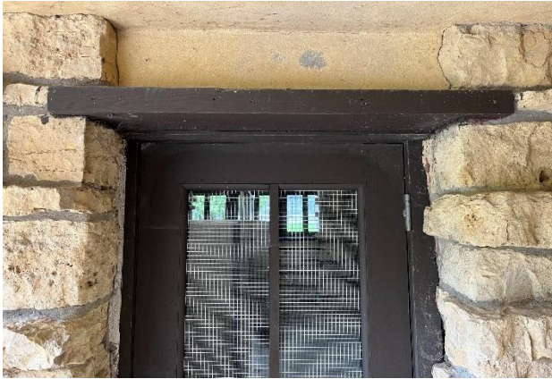
Figure 102. Non-original restroom door with wood lintel bearing on stone.
