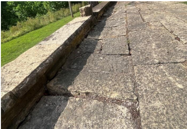
Figure 64. The stone paving and parapet wall adjacent to the coping unit are displaced and partially collapsed.
