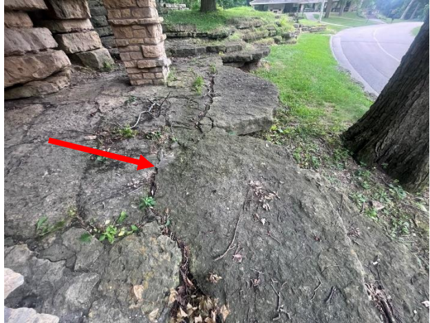
Figure 457. Displaced stone unit, sloped away from the terrace.
