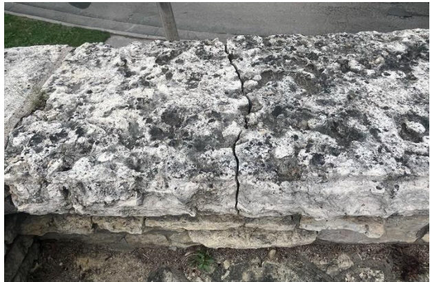
Figure 459. Cracking at coping unit.
