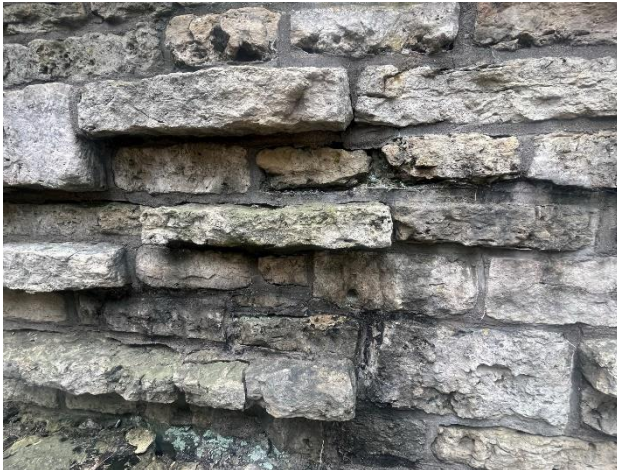
Figure 476. Black-colored soiling at the stone units at the cheek wall for the east stair.
