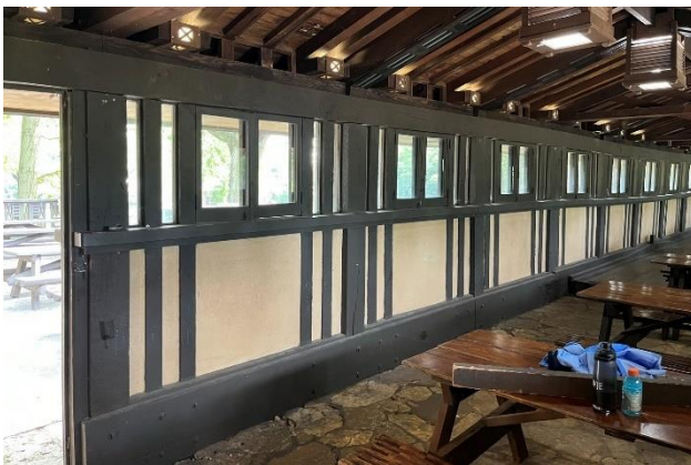
Figure 321. Interior view of wood-framed stucco walls as viewed from bridge.
