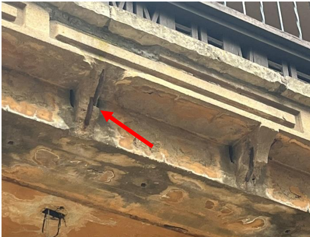
Figure 483. Spall at concrete bracket at balcony.
