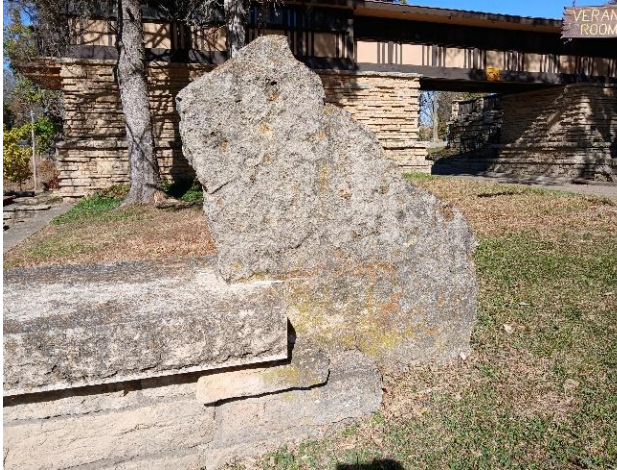
Figure 43. Detail of stone at end of the stepped parapet wall.
