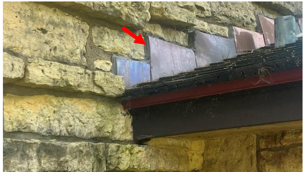
Figure 111. Copper flashing at restroom wing, set in sealant.
