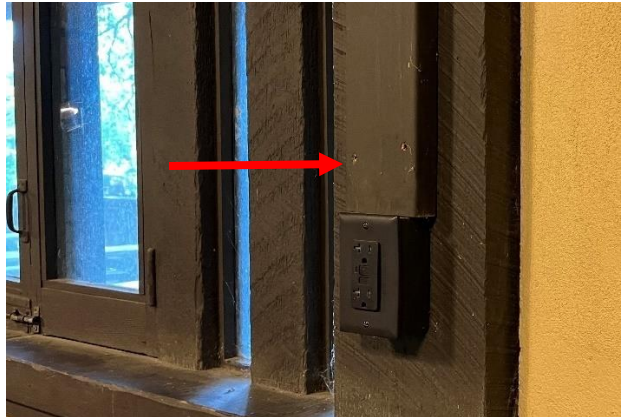
Figure 438. Non-original outlet with wood 2x4 concealing the surface-mounted conduit.
