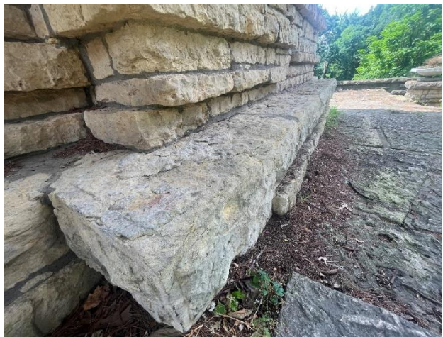
Figure 80. Rock-faced finish stone watertable unit.
