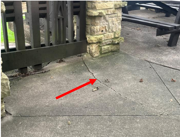
Figure 479. Cracking at the concrete paving of the south terrace.
