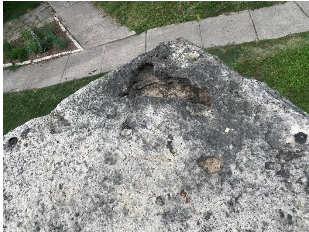
Figure 477. Large divot in stone at coping unit.
