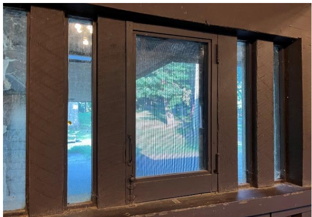
Figure 335. Interior view of single sash casement window.
