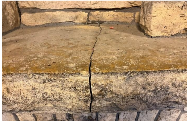
Figure 465. Cracking at mantel of east room fireplace.
