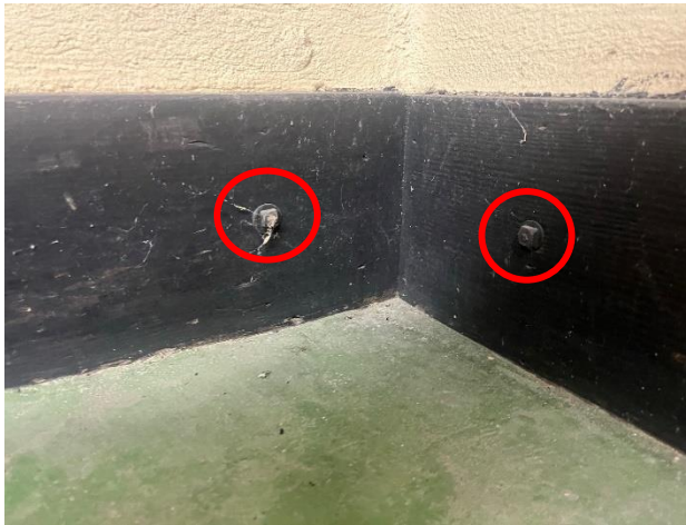
Figure 269. Washer and nut at the end of the bolt visible at the interior.
