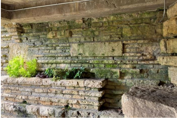
Figure 474. Biological growth above the planter box at the covered stone terrace.
