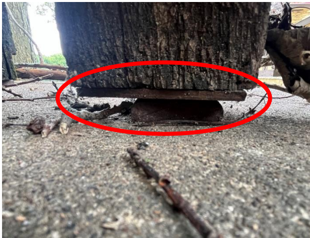
Figure 505. Surface corrosion at a steel plate that supports a wood post for the terrace guard rail.
