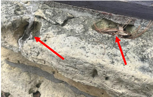
Figure 190. Deep pockets and pits in the stone.
