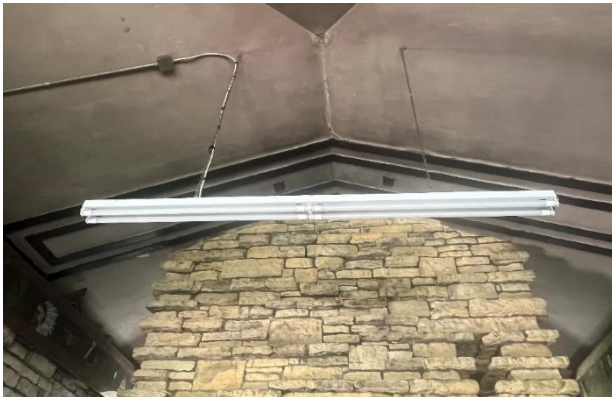
Figure 173. Non-original double ballast fluorescent light fixture suspended from the ceiling at the community room.
