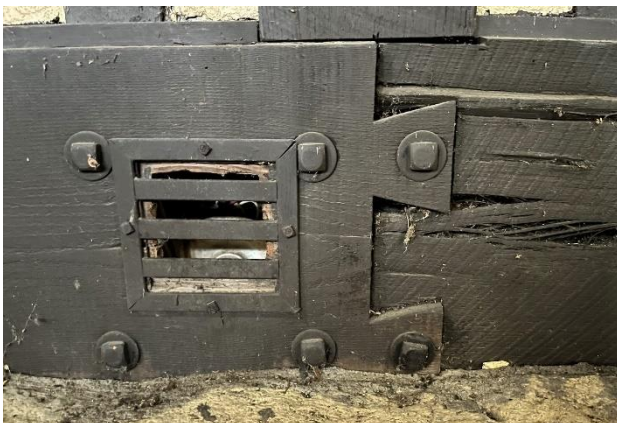
Figure 407. Dovetail connection between framing members.
