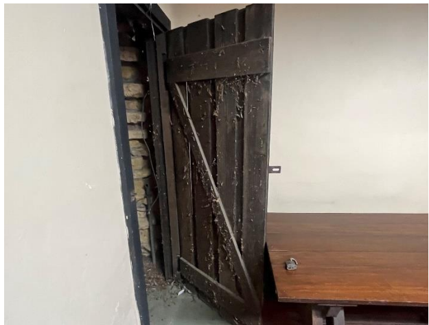
Figure 274. Horizontal and diagonal bracing on the interior face of the door.
