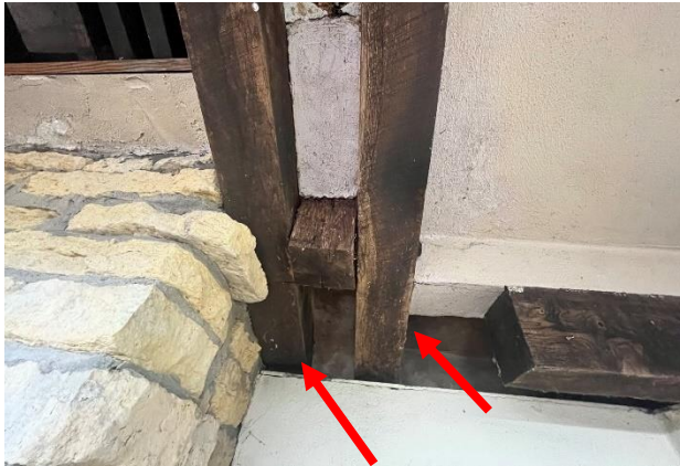
Figure 235. Ends of wood framing members for dormer roof.
