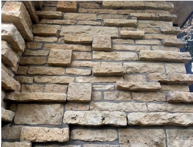
Figure 77. Random stone coursing and projecting stone units at exterior walls.
