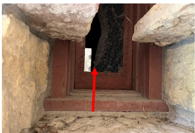
Figure 218. Displaced metal screening at wood-framed window.
