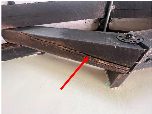
Figure 315. Crack extending the full length at the underside of diagonal bracing member.
