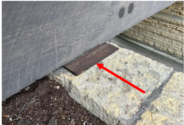
Figure 406. Steel plate upon which the bridge deck framing bares.
