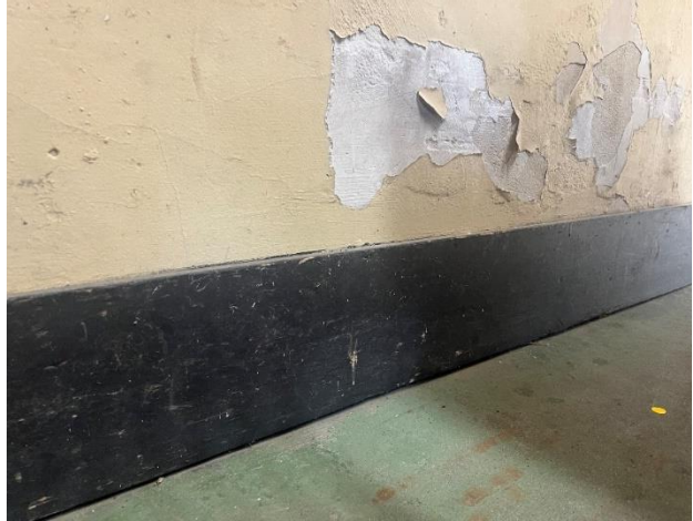
Figure 272. Wood baseboard without projecting wood trim above.
