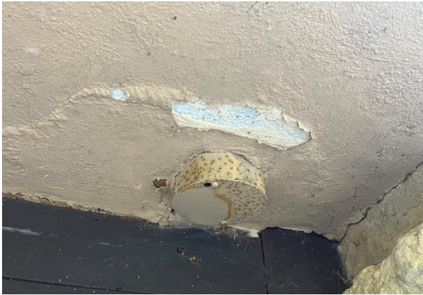
Figure 285. Exterior surface-mounted junction box near the south entrance door.
