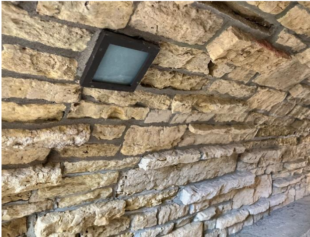
Figure 370. Stone coursing at the arch.
