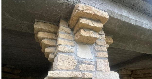
Figure 363. Stone dutchman at pier to replace abandoned light fixture.
