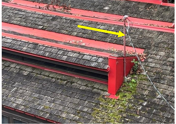
Figure 286. Conduit for main service line located at the north end of the east dormer.
