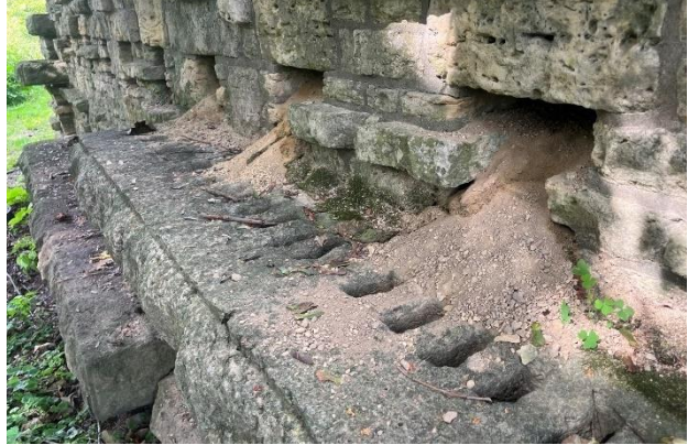
Figure 67. Piles of sand washout were observed at ports in the terrace wall adjacent to the displaced paving.
