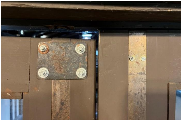
Figure 491. Door leaf out of plumb near area of displaced roof framing.
