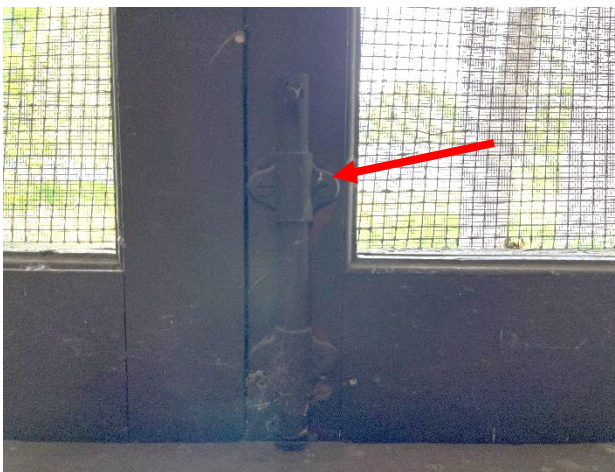
Figure 91. Vertical slide lock extending into a pocket in the sill.
