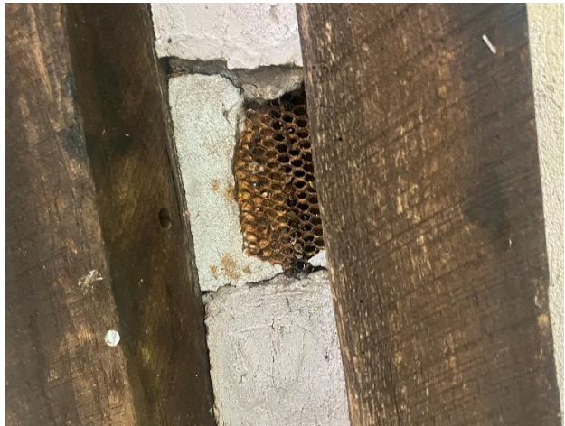
Figure 324. Area of damaged plaster with metal lath exposed.
