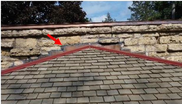
Figure 110. Copper flashing at stone chimney.
