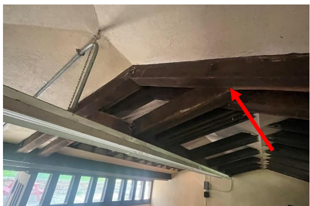
Figure 234. Wood roof framing at dormers.
