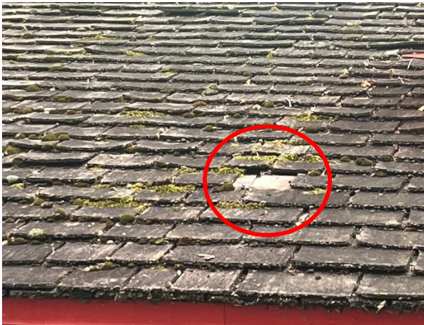
Figure 321. Missing roof shingle.
