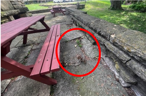
Figure 66. Displaced stone paving at Veranda Rooms terrace.
