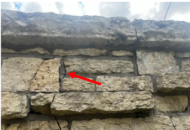
Figure 460. Cracking at stone wall that extended from coping.
