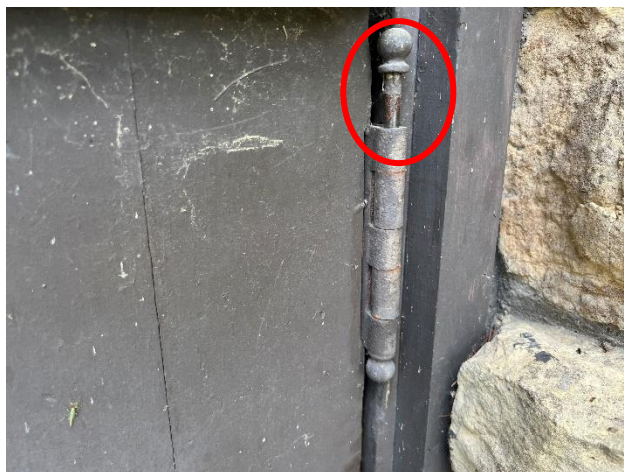
Figure 220. Displaced hinge at door.
