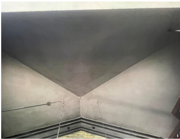
Figure 133. Plaster ceilings following the hip roof form of the roof.
