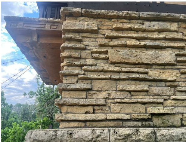
Figure 317. Typical stone cladding at Bridge Complex.
