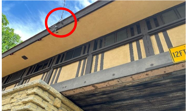
Figure 432. Main utility line attached to wood fascia at north elevation of bridge.
