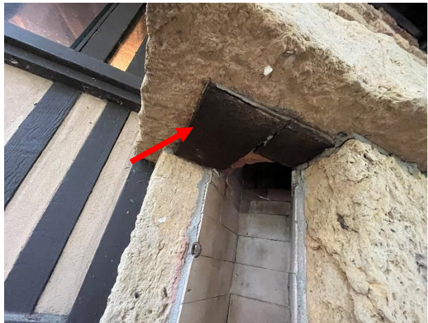
Figure 421. A 6 inch steel plates supporting stone unit above.
