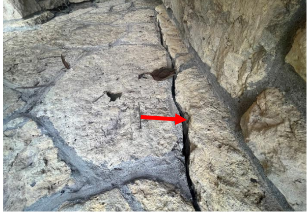
Figure 189. Open joint between the stone paving at the recessed restroom vestibule and at the adjacent restroom enclosure.
