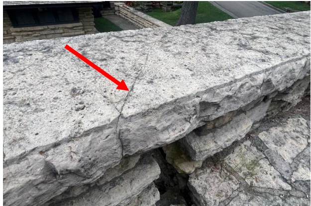
Figure 471. Cracking at the upward-facing surface of a ledge unit.
