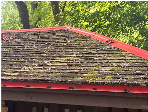
Figure 322. Biological growth and moss on the wood shingles.
