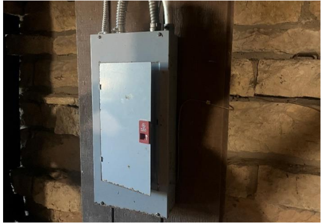
Figure 172. 120-amp, 120/240-volt electrical panel, located in the mechanical room.
