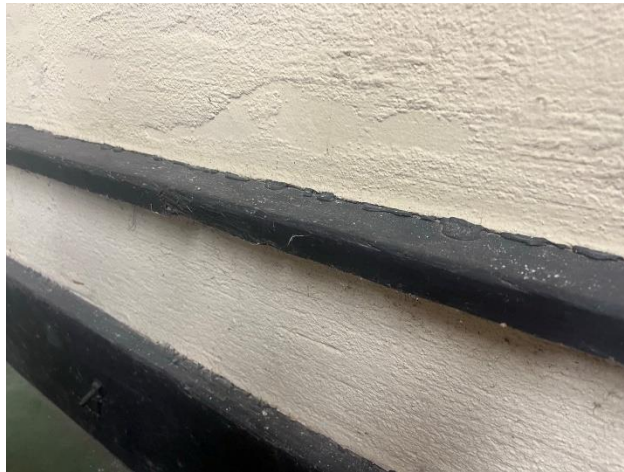
Figure 270. Projecting wood trim piece positioned above the baseboard.
