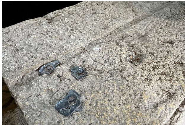
Figure 429. Embedded anchors and routed channel in stone indicate a previously installed screen feature on stone.
