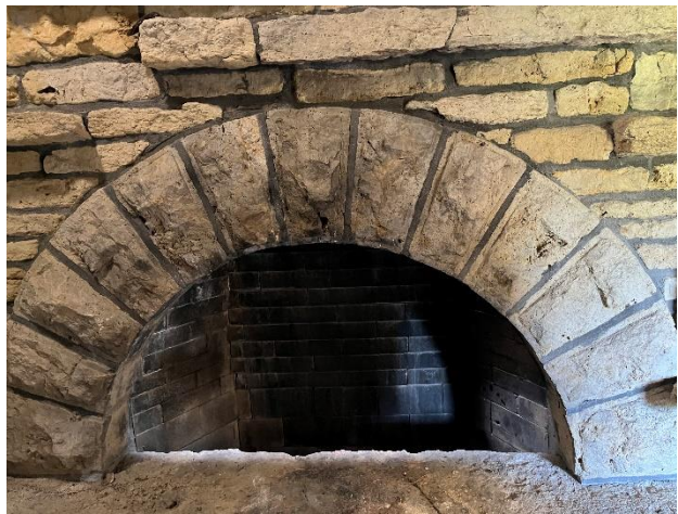
Figure 151. Load-bearing arched opening with expressed stone voussoirs.
