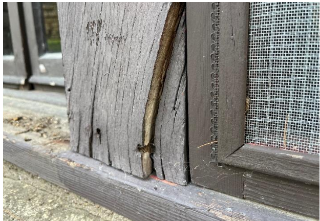
Figure 212. Split at the wood cladding of window mullion that extends the full depth of the wood for a length of approximately 6 inches.
