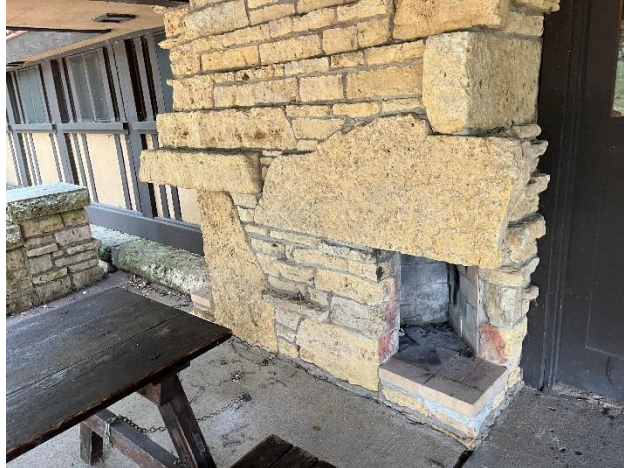
Figure 419. Large face bed stone above north firebox.
