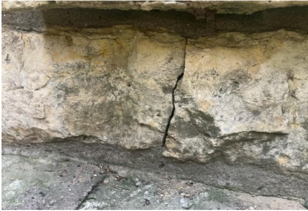
Figure 182. Localized vertical cracking at the center of several field of wall stone units.
