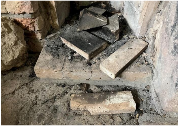
Figure 468. Four of the upper brick units that are loose.
