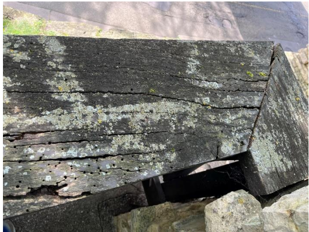
Figure 502. Severe deterioration and biological growth at wood of top rail of railing.
