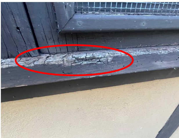
Figure 339. Distress at the top surface of a window sill.
