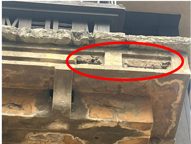
Figure 484. Spall of concrete at balcony edge.
