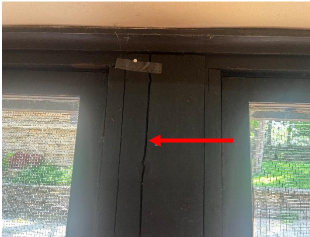
Figure 314. Vertical split at the interior side of the wood post.
