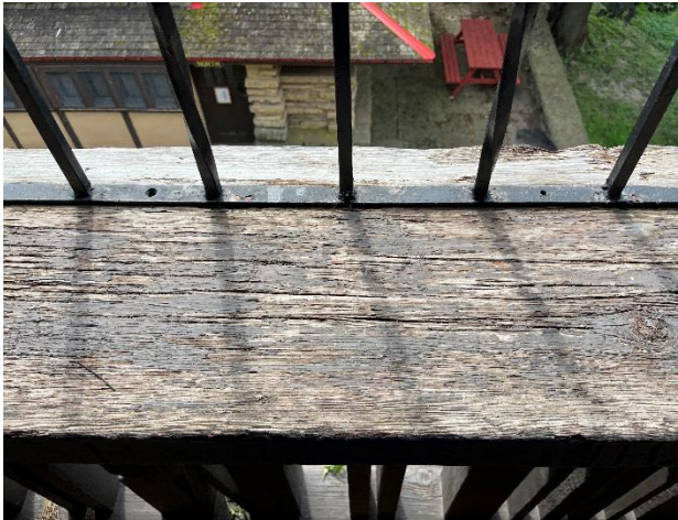
Figure 499. Deterioration at wood top rail of balcony guardrail.
