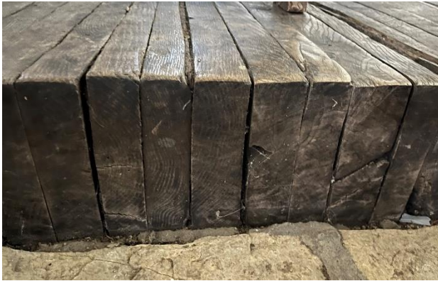
Figure 403. Ends of wood deck framing members.
