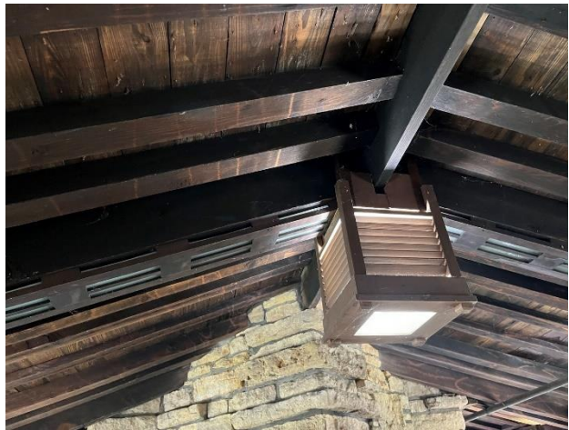
Figure 325. Roof framing with wood-framed frosted glazing screen at bridge roof.
