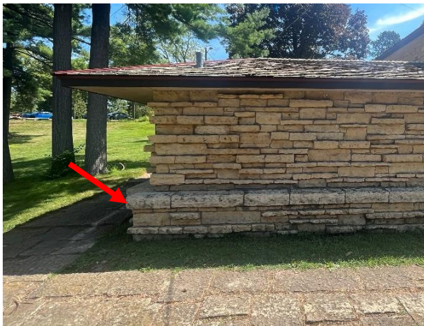
Figure 79. Stone watertable at base of building elevation.
