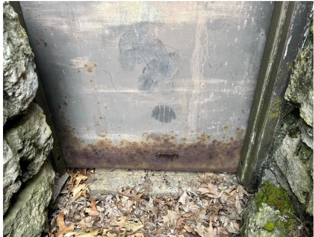
Figure 517. Corrosion along the bottom of the door leaf.
