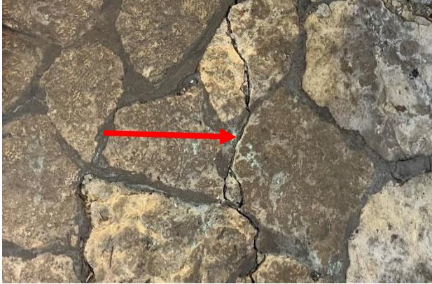
Figure 462. Cracking at stone floor pavers.
