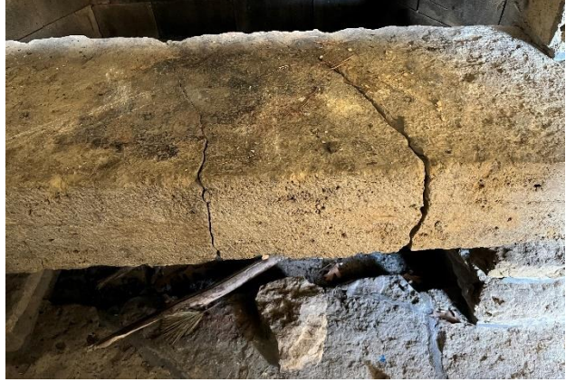
Figure 183. Significant vertical cracking at upper fireplace mantel.
