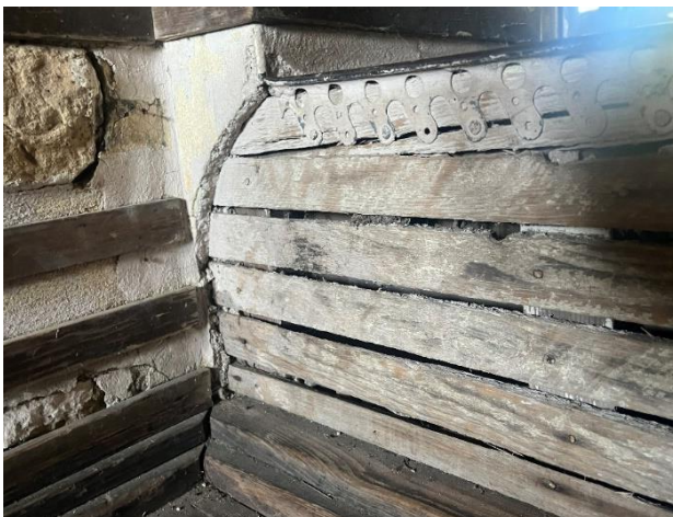
Figure 206. Exposed wood lath and edge beads.
