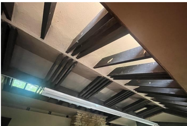
Figure 233. Portions of the rafters and diagonal bracing members visible at the building interior.
