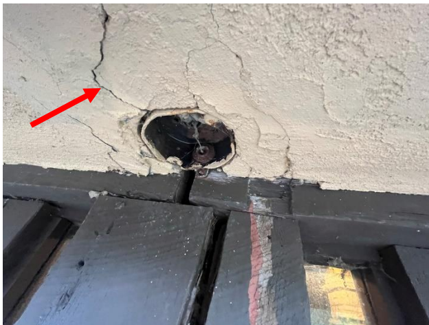
Figure 507. Abandoned junction box in the soffit has resulted in cracking of the adjacent stucco.
