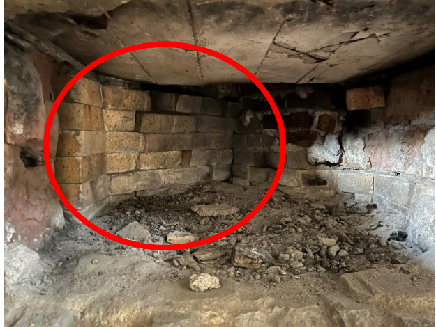
Figure 482. Displaced and loose brick cladding at the firebox.
