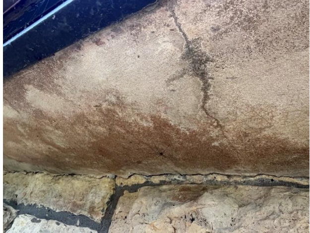
Figure 209. Discoloration of stucco adjacent to crack, indicating that moisture or water infiltration may have been associated with the crack at one time.
