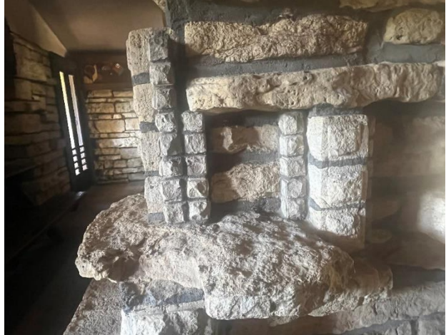
Figure 155. A series of stacked small and large square stone units at the southwest corner of the chimney.
