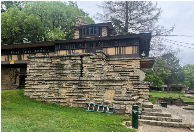
Figure 383. North elevation of the west stair cheek wall. Note that the wall construction includes the watertable and copings present at the walls.
