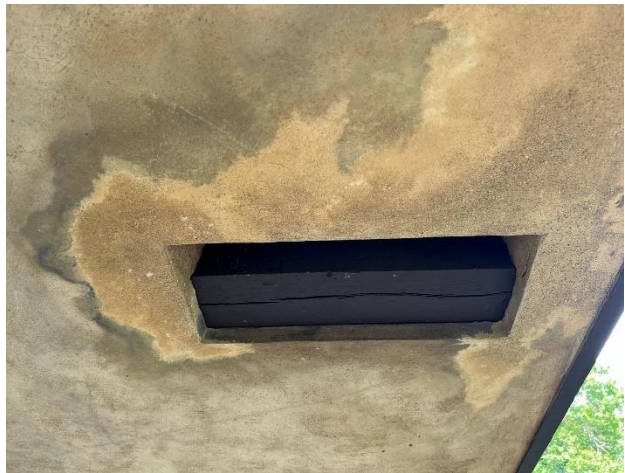
Figure 262. Pocket in roof eave.
