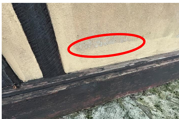
Figure 514. Failed paint at stucco wall exposing the white underlying stucco.
