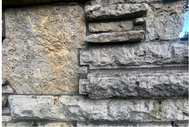
Figure 384. Carved dovetailed detail at ends of stone units.
