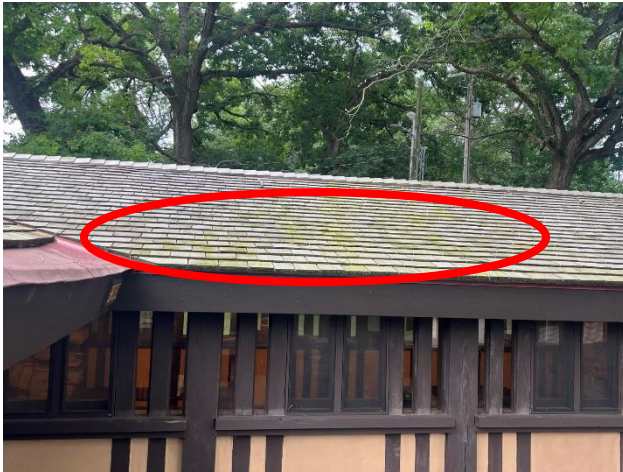
Figure 508. Mild biological growth at the west-facing slope of the roof.
