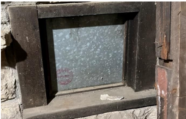
Figure 97. A removed sash infilled with non-original galvanized metal panel.
