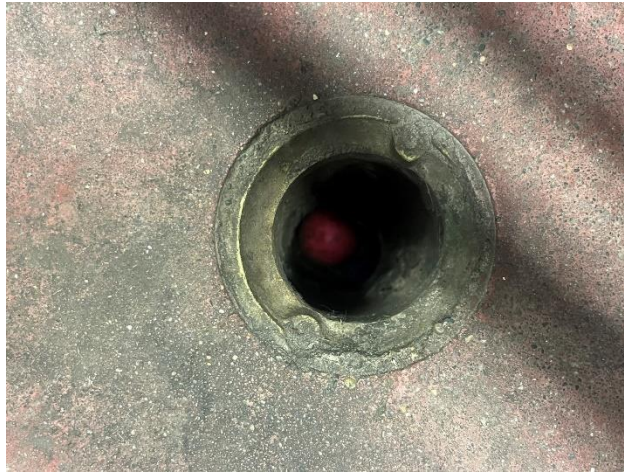
Figure 307. Missing drain cover.
