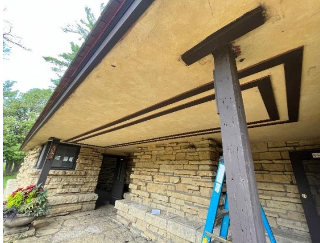
Figure 118. Wood trim at soffit of recessed vestibule.
