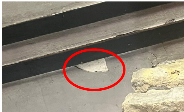
Figure 205. Debonded plaster finish that has fallen loose.
