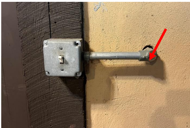
Figure 513. Untreated penetration with gap between conduit and stucco.
