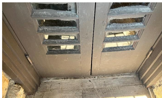
Figure 106. A wood threshold separates the interior from the exterior.
