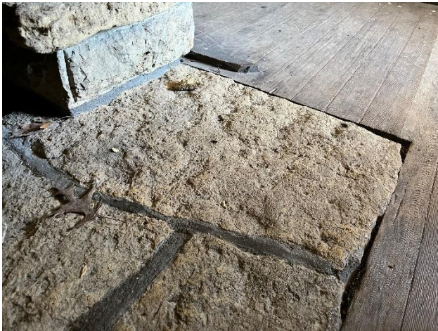
Figure 156. Stone hearth flush with the wood flooring.
