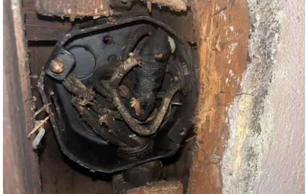
Figure 166. Junction boxes set in the plaster finish of the walls and ceiling.
