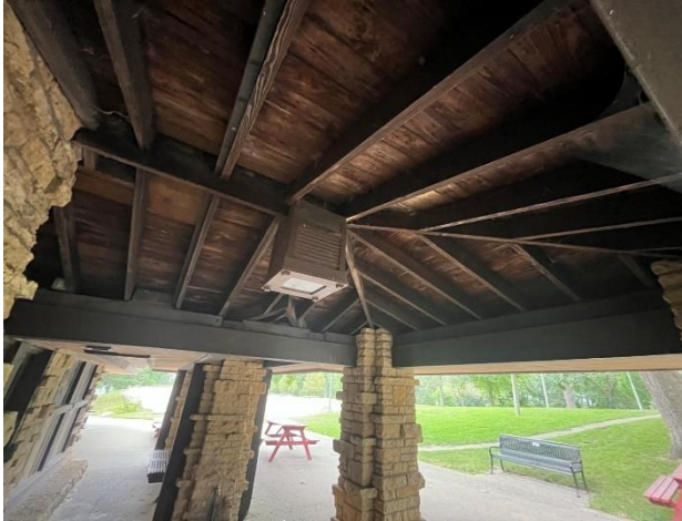
Figure 322. Roof framing at east entrance vestibule roofs.
