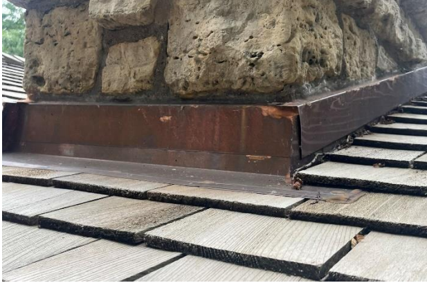
Figure 354. Copper flashings in the mortar joints.
