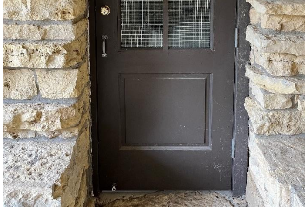
Figure 103. Faux recessed panel at the lower half of the door.
