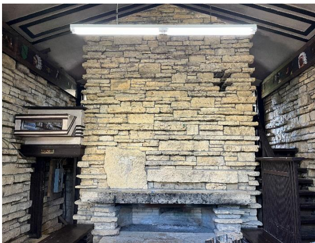
Figure 146. Large stone chimney extending two-stories.
