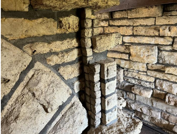
Figure 154. Small and large stacked square stone units.
