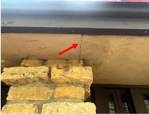
Figure 328. Crack near corner of a stone pier where the depth of the soffit changes.
