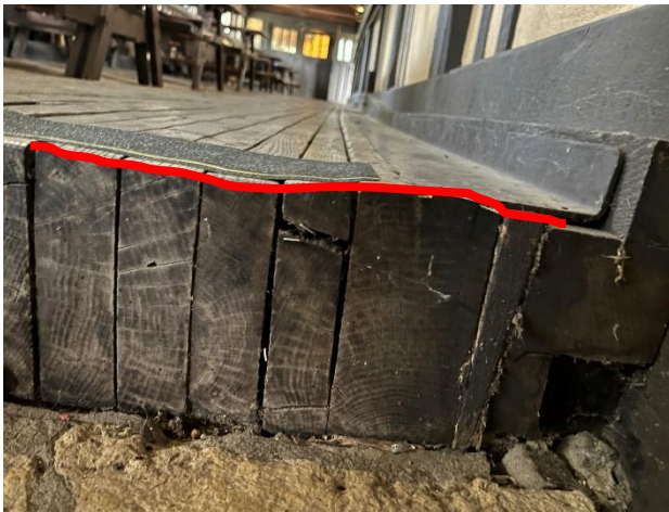
Figure 497. Irregular bridge deck surface and localized crowned area.
