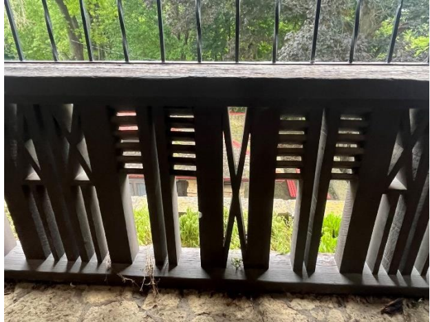
Figure 359. Original wood railing sitting on stone pavers.
