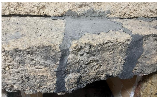
Figure 294. Previously repaired crack.
