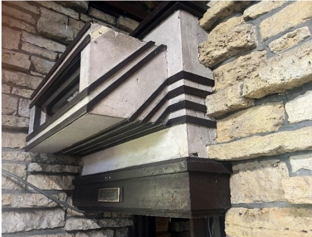
Figure 128. Wood trim bands extend horizontally and diagonally across the plaster balcony walls.
