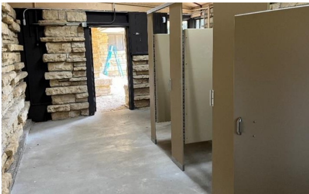
Figure 125. Polished concrete flooring in restrooms.
