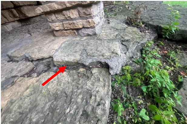
Figure 458. Displacement of stone pavers adjacent to concrete footing for pier.
