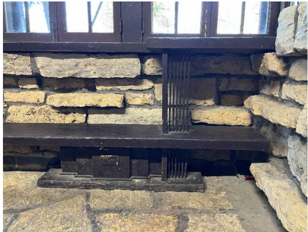
Figure 158. Sturdy wood supports on either end of the bench seat.
