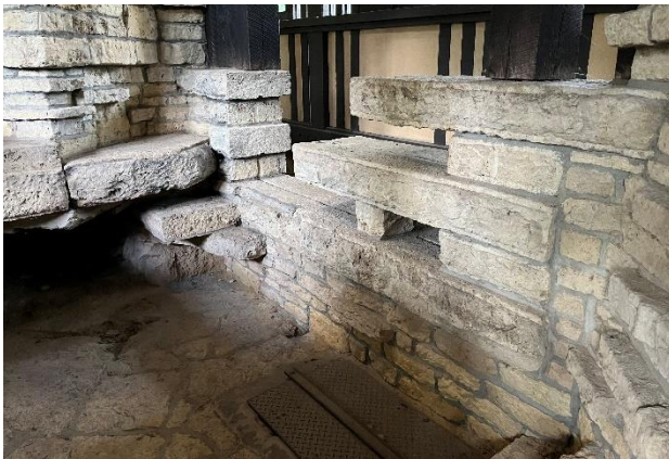
Figure 428. Alternating long and short stone units at south knee wall.
