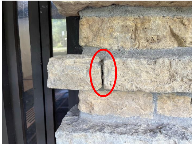
Figure 304. Open horizontal mortar joint.
