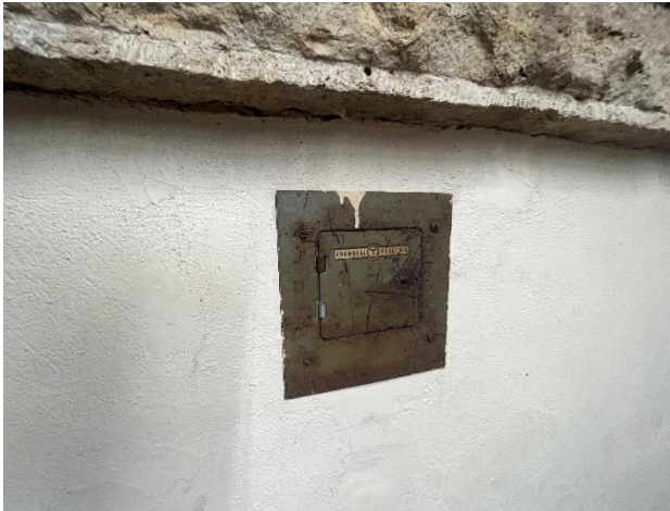
Figure 277. Original Trumbell Electric box set within the plaster wall.
