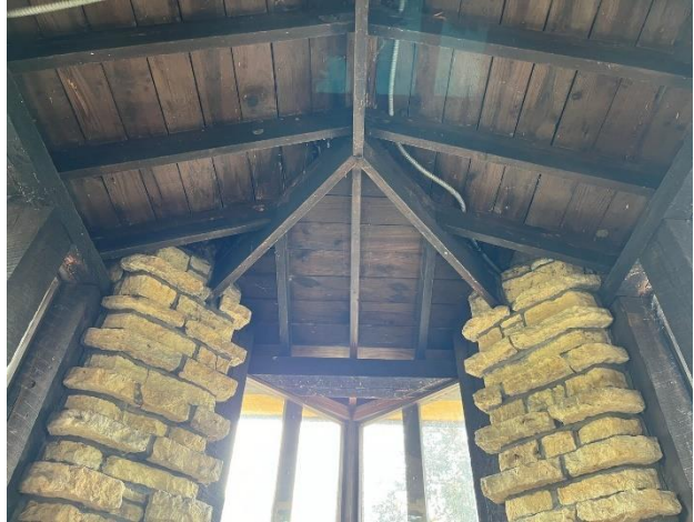
Figure 323. Roof framing at lookout tower roof.
