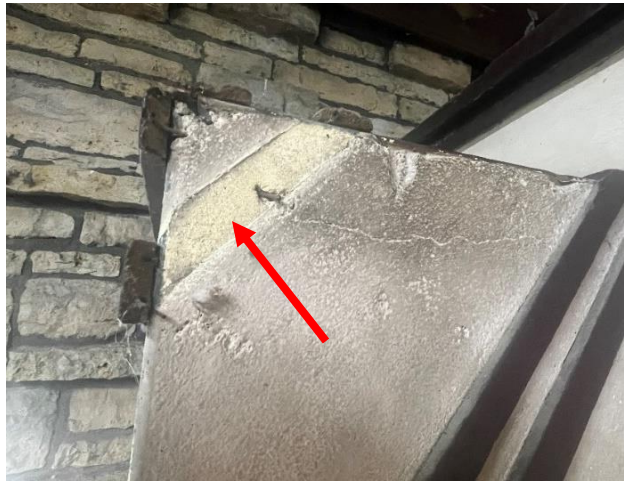
Figure 195. Missing wood trim at the plaster walls.
