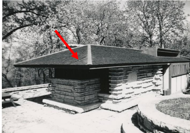
Figure 29. South elevation of the Veranda Rooms, circa 1973 (Source: Center for Dubuque History) The electrical posts that receive the main utility line have been removed. Repairs are visible in the shingle roofing where the posts were located (arrow)
