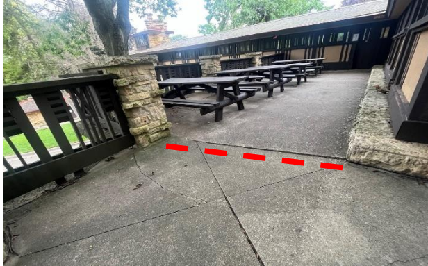
Figure 372. Concrete paving at the south terrace. Note that concrete in the foreground is different than the concrete in the background.
