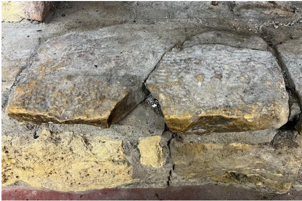
Figure 297. Cracked and loose stone at the hearth of the north fireplace.
