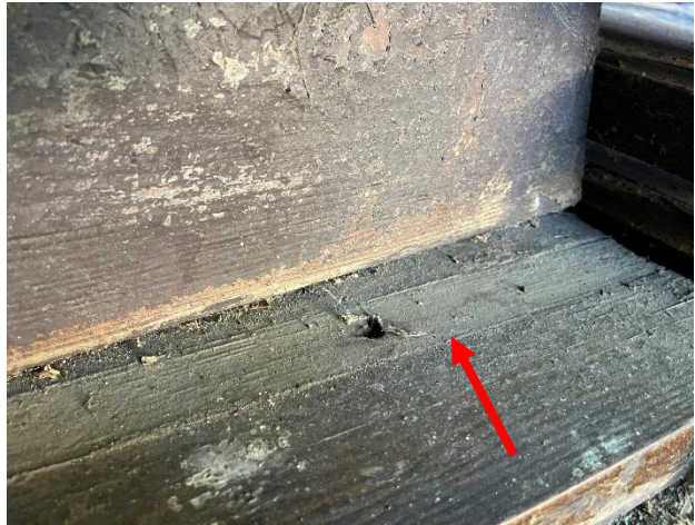
Figure 197. Displaced vertical board that supports the center of the bench seat.
