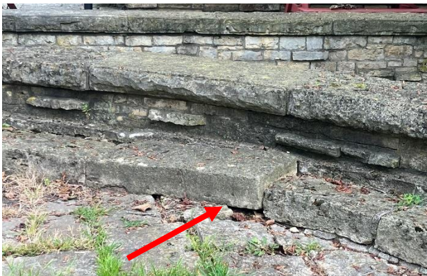
Figure 70. A few stone units at the semicircular terrace seating areas are displaced or heaved.
