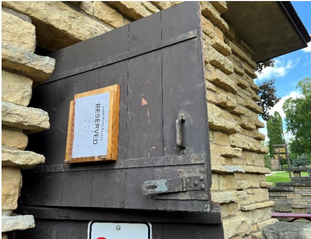
Figure 100. The upper leaf of the south door is reinforced with non-original metal straps that span horizontally across the leaf.
