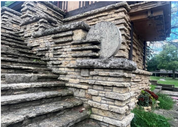
Figure 385. There is a carved circular stone unit mounted onto the stepped coping units at the south side of the stairs.
