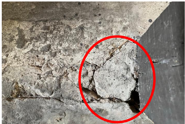
Figure 486. Crack and spall at concrete flooring of north annex.
