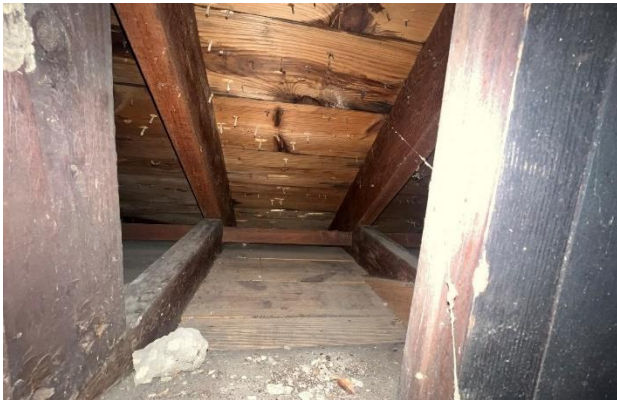
Figure 231. Eave framing at wood roof soffit.
