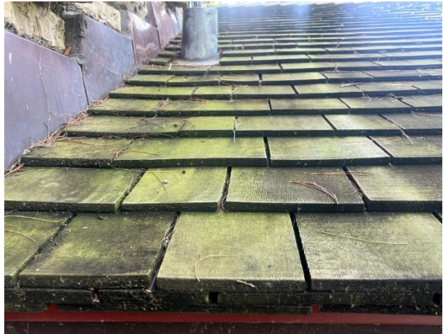
Figure 201. Biological growth at wood shingles.
