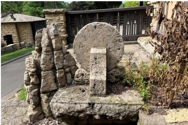
Figure 389. Stone cheek wall that features a circular stone decorative unit mounted onto the coping and the remains of what appears to be a light fixture integrated into the stone base.
