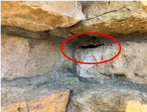
Figure 305. Spalled stone along the edge of a mortar joint, resulting in a partially open joint.
