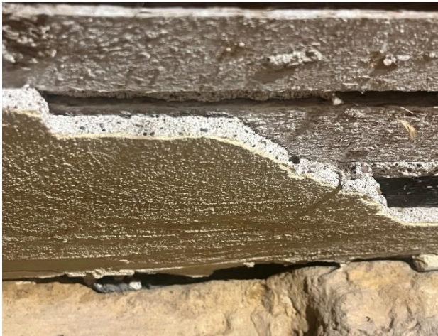
Figure 137. Remaining 3/8-inch-thick plaster with a yellow/beige finish coat.
