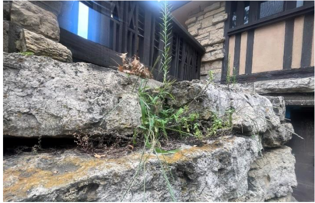
Figure 61. The voids measured as much as 6 inches wide and to a depth of a few feet. Plants were growing within some of the voids.
