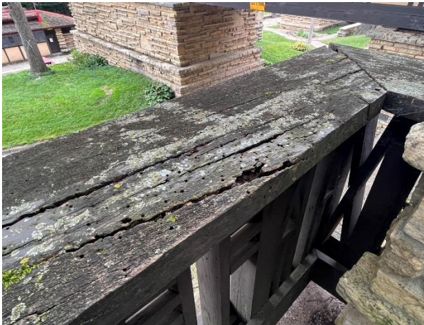
Figure 501. Severe deterioration and biological growth at wood of top rail of railing.
