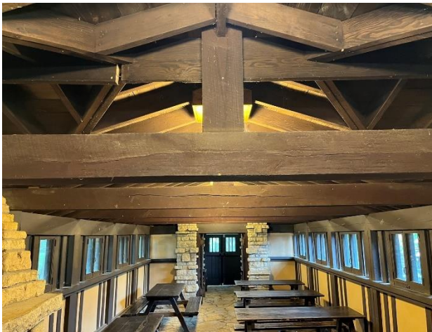
Figure 324. Roof framing at east room.
