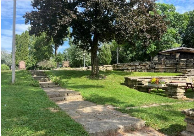
Figure 47. The steps vary in the depth of the treads but are typically 4 to 6 inches tall.
