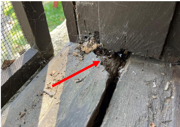
Figure 211. Split wood sill that was soft when probed.
