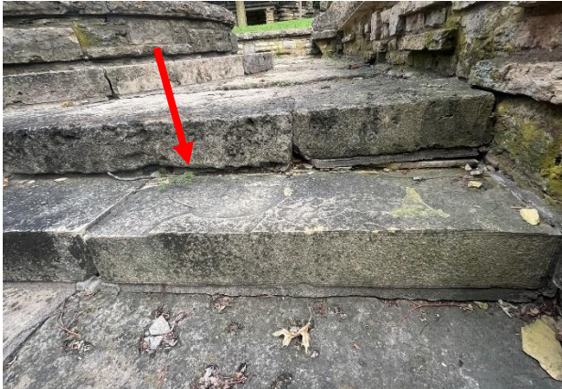
Figure 68. Open mortar joints at stone stair treads.
