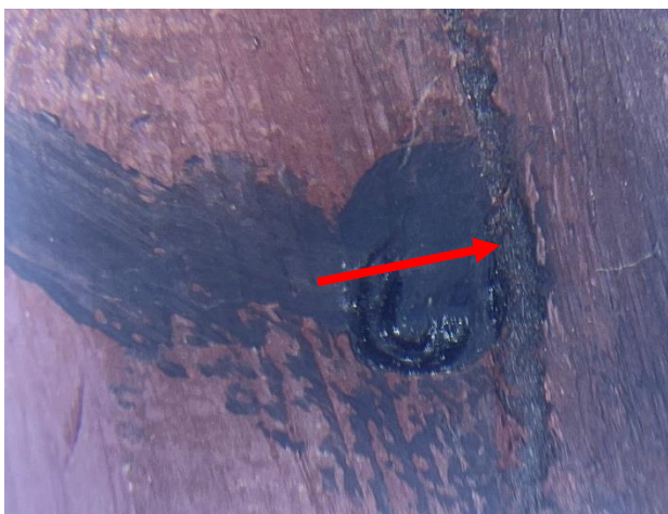
Figure 223. Scratch extended through the painted surface and abrading the paint coating.
