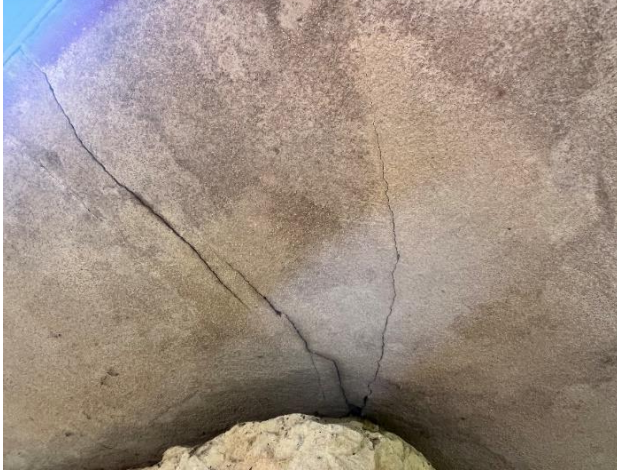
Figure 208. Cracking at the underside of the stucco soffit.
