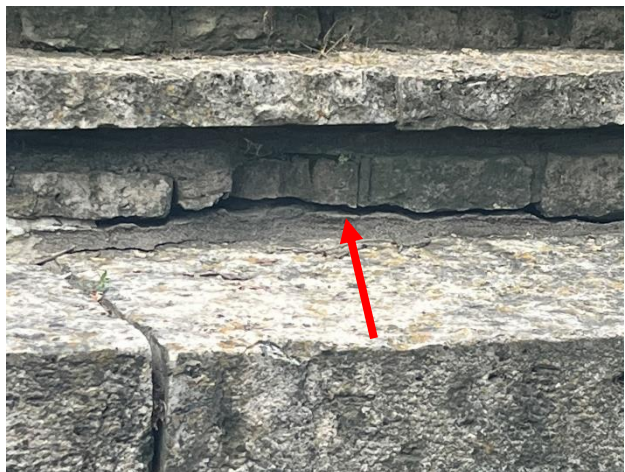
Figure 473. Cracking at the mortar joint between a stone-paved stair tread and the stone-clad face of the stair rise.
