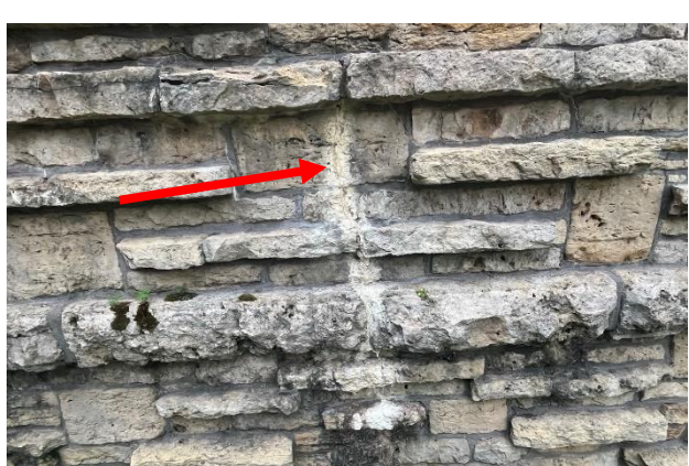
Figure 461. Efflorescence at lower portion of a vertical crack.
