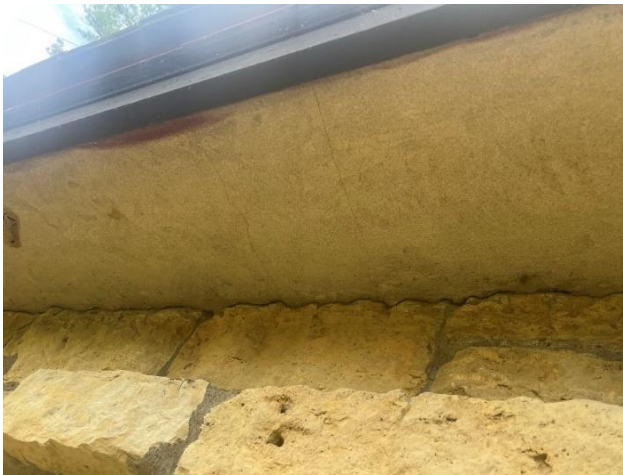
Figure 114. Stucco at overhanging eaves.
