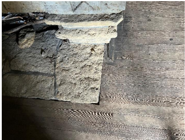
Figure 124. Tongue-and-groove wood boards at upper overlook level.
