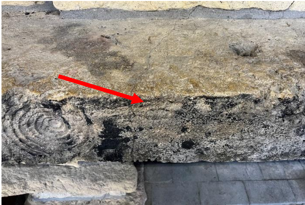
Figure 184. Vertical cracking at lower fireplace stone mantel.
