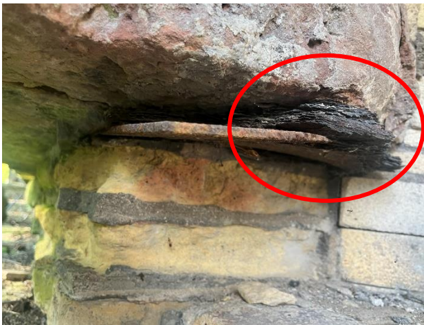
Figure 317. Corrosion and rust jacking at steel plate at fireplace.
