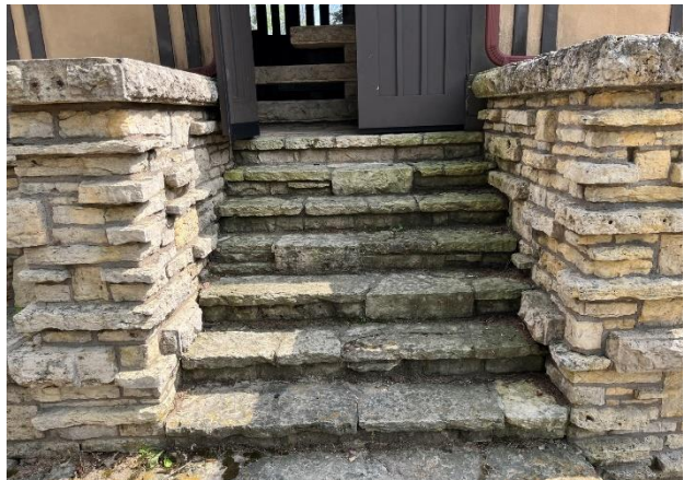
Figure 386. Stone stair treads at upper flight of west stair.
