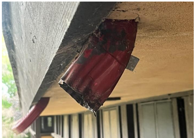
Figure 353. Red aluminum downspout.
