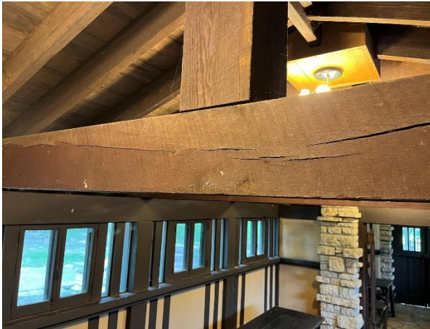
Figure 495. Splits along the center of a roof beam that spans across the east room.
