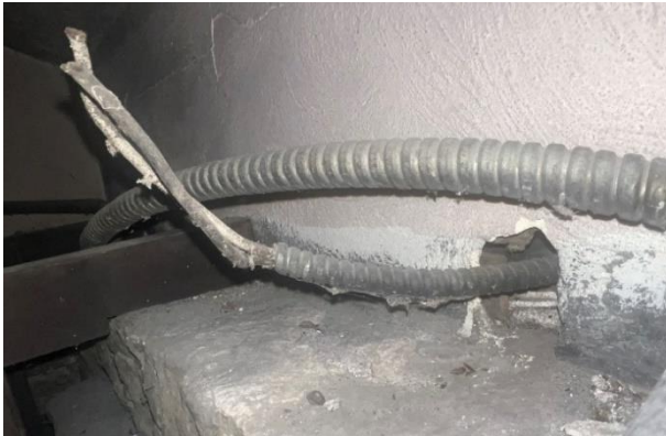
Figure 165. Coiled flexible metal conduit.
