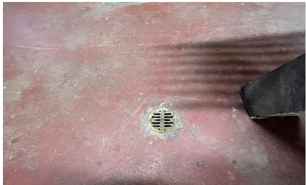
Figure 267. Floor drain.
