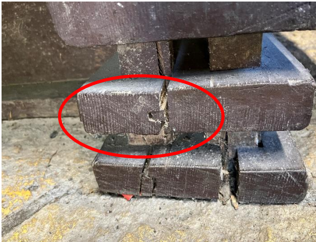
Figure 198. Split decorative 2x8 wood members that surround the support posts at the base of the bench.
