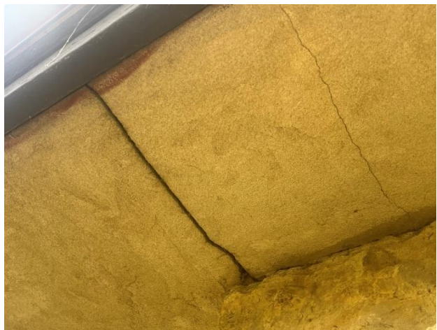
Figure 207. Cracking at the underside of the stucco soffit.
