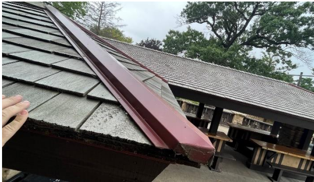
Figure 350. Ends capped with sheet metal.
