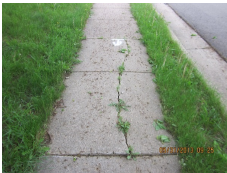
Cracked and heaving sidewalk - Tripping hazard
