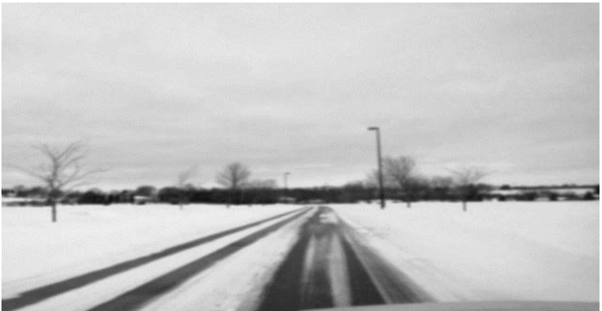
Pavement fully plowed with driving lanes treated:
