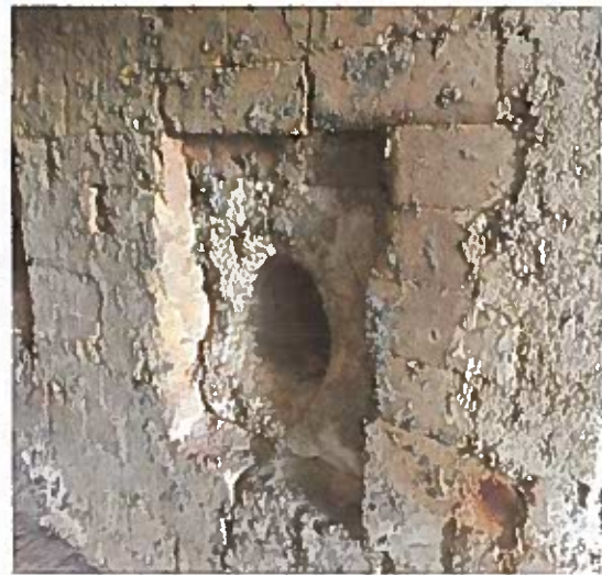
Sample R-2: Refractory brick and mortar, taken from front right side of furnace.
