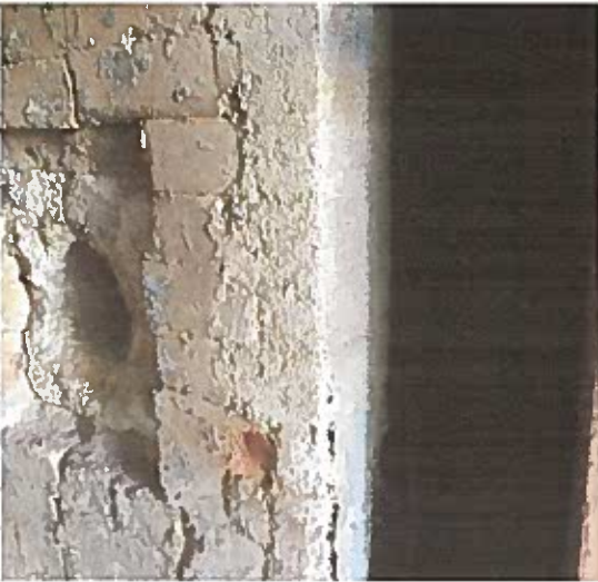
Sample R-1: Taken from front Right Corner, replacement refractory cement.
