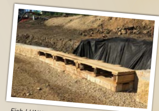
Fish LUNKERS were installed along the edge of the creek in multiple locations.
