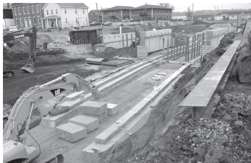
Limestone blocks line the creek channel.
