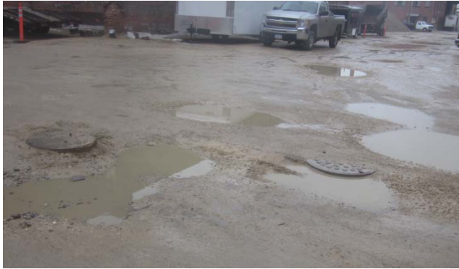
Photo 4: Impervious, Flood-prone Historic Millwork District Street Prior to Federal TIGER Grant Complete Streets Improvement Project
