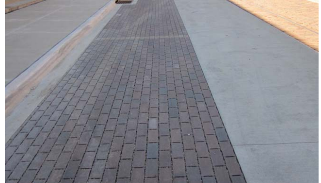
Photo 5: Historic Millwork District Pervious Pavement System that Conveys Stormwater into the Underlying Soil
