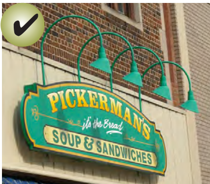
Direct lighting at signage from an external, shielded lamp.
