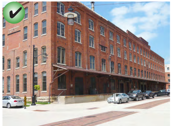
After: A parapet wall, loading docks, and canopies should not be altered, especially those on primary facades, or when they are highly visible.
