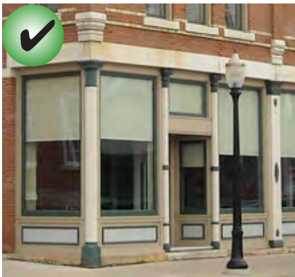
A kickplate, located below the display window adds interesting detail to the streetscape and should be preserved.
