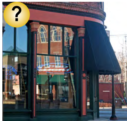
The installation of this canopy is generally acceptable; however, a better approach is to locate the canopy to fit within the wall opening.
