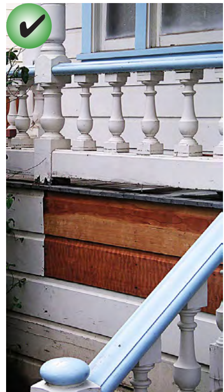
Replace only the amount required. If a few boards are damaged beyond repair, then only they should be replaced, not the entire wall.
