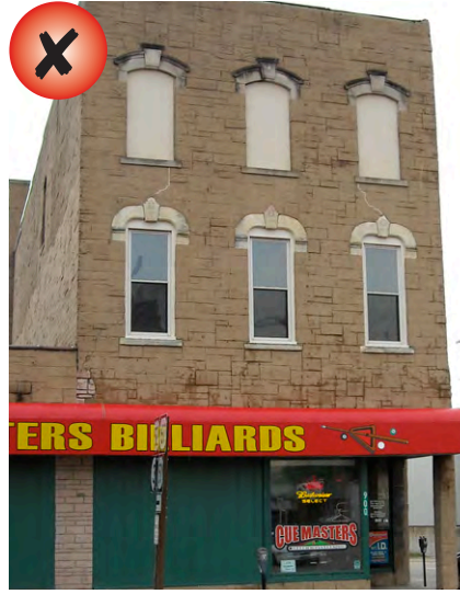
Inappropriate treatment on upper story windows
