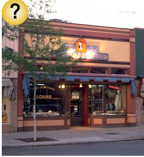
Interim improvements to the building included removing the canopy, providing a new sign and painting the stucco covering.
