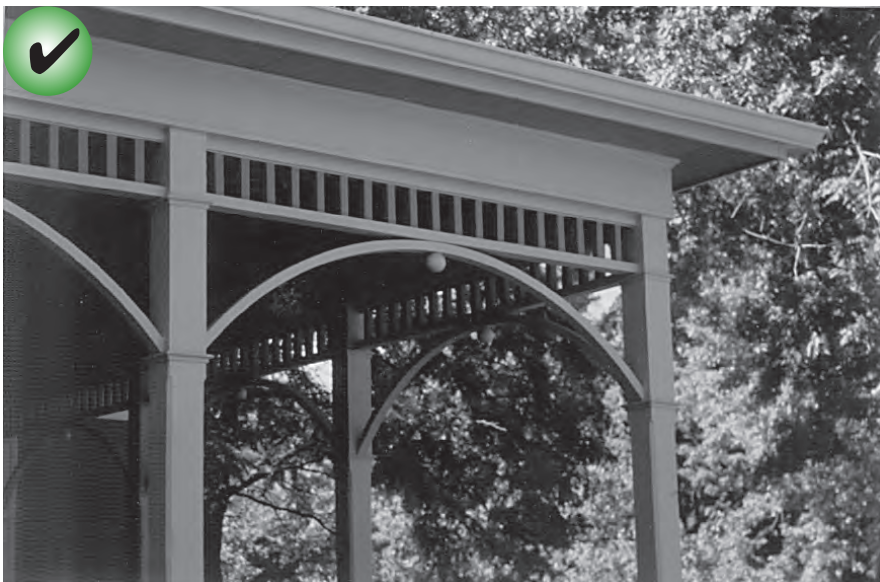
When reconstruction of an element is impossible, develop a new design that is a simplified interpretation of it.
