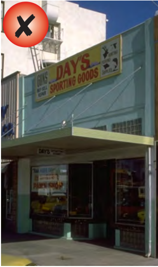
Original building remodel with stucco covering.
