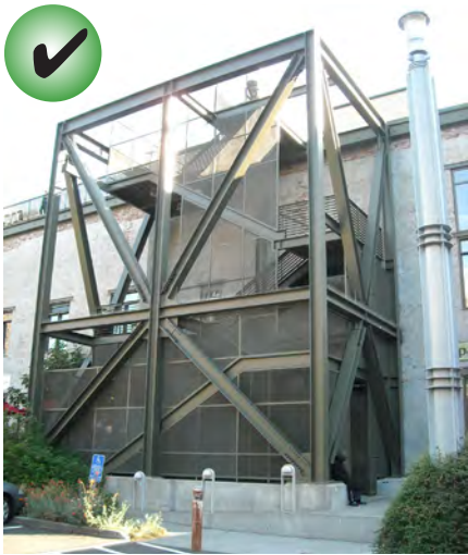
A contemporary interpretation of a fire escape is an appropriate addition to the rear or secondary facade of a historic building.
