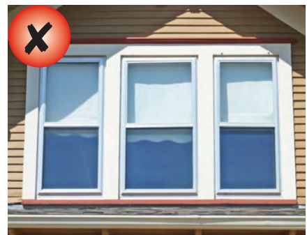
Unfinished metal storm windows such as these alter the character of window openings, and should not be used on primary elevations. A metal storm window may be appropriate if the frame matches the proportions and profiles of the original window and has a painted finish.
