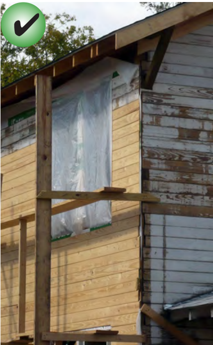
Match the original material in composition, scale and finish when replacing materials on primary surfaces.
