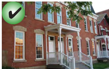
After: Reconstructed porch and new windows installed in original openings
