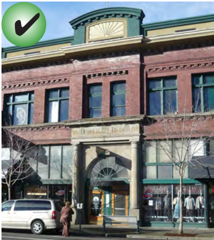
After: Cornice reconstructed using material similar to the original.
