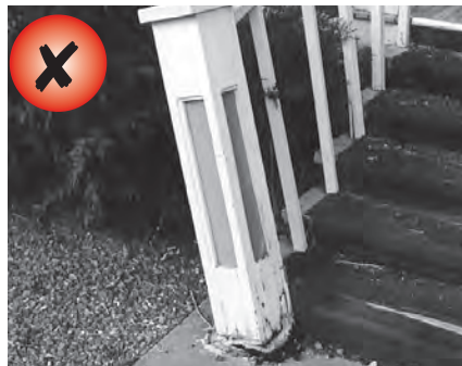
Before: A deteriorated railing should be repaired rather than replaced.
