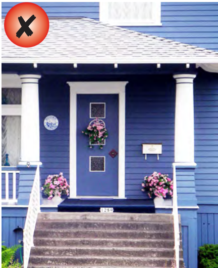
A new door such as this, that differs from the original or that is inconsistent with the historic style, is inappropriate on a primary wall.
