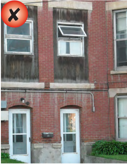
Inappropriate reduction in window size
