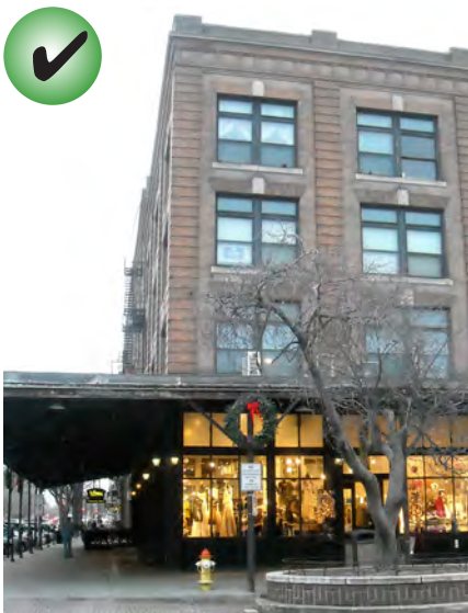
Transoms, the upper glass band on door openings, introduced light into the depths of the building, saving on light costs. These bands should not be removed or enclosed.
