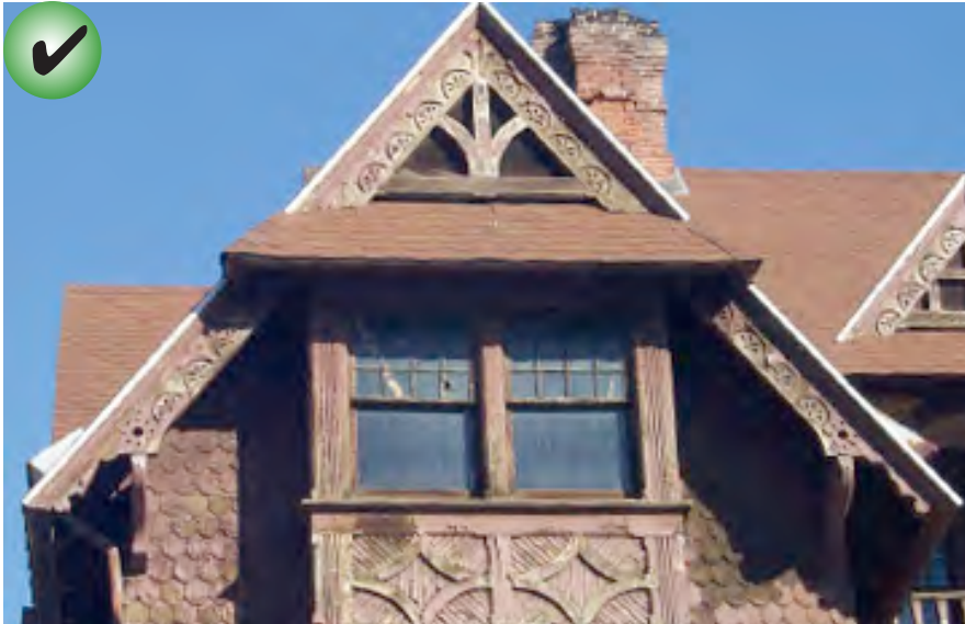
Carved bargeboard and spandrel panels on the gable end of a Stick style house are key architectural details that should be preserved.
