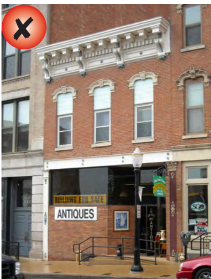
Inappropriate reduction in upper story windows and storefront modification
