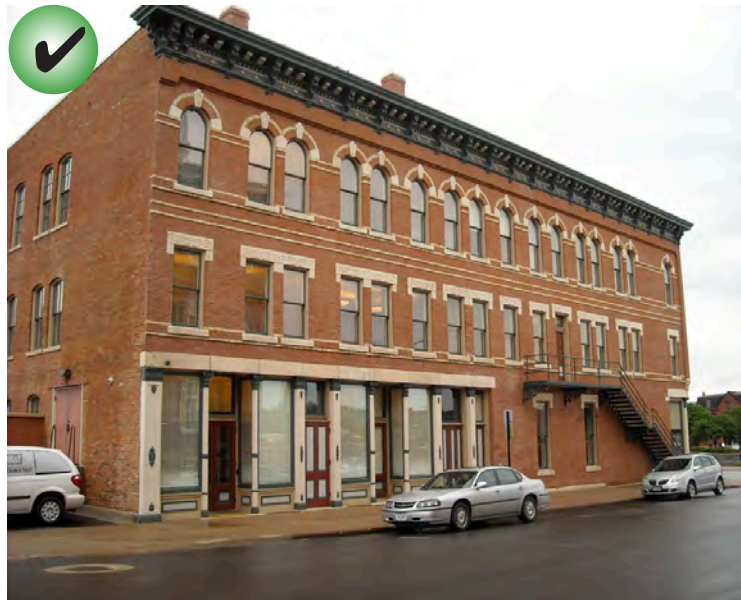
The new fire escape is appropriately located on the secondary facade and is also a good representation of a compatible design.
