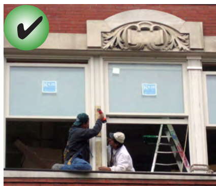
Match the appearance of the original window design (i.e., if the original is double-hung, use a double-hung replacement window, or a window that appears to be double-hung).
