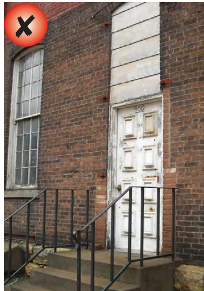
Inappropriate door and transom replacement
