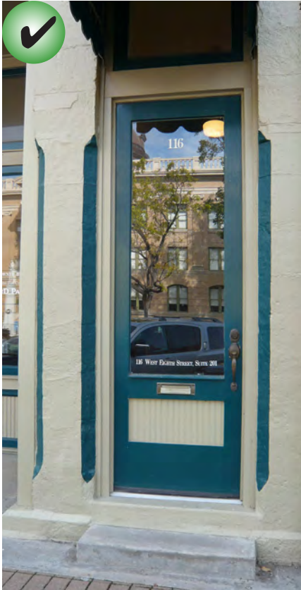
When replacing a door, use materials that appear similar to that of the original.
