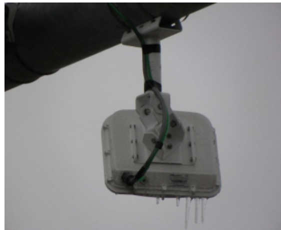
Closeup of a microwave traffic detector
