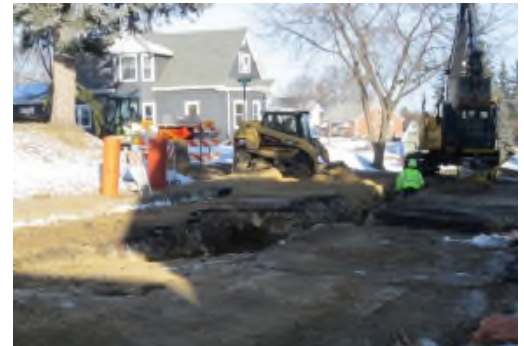
Emergency Water main repair in the winter
