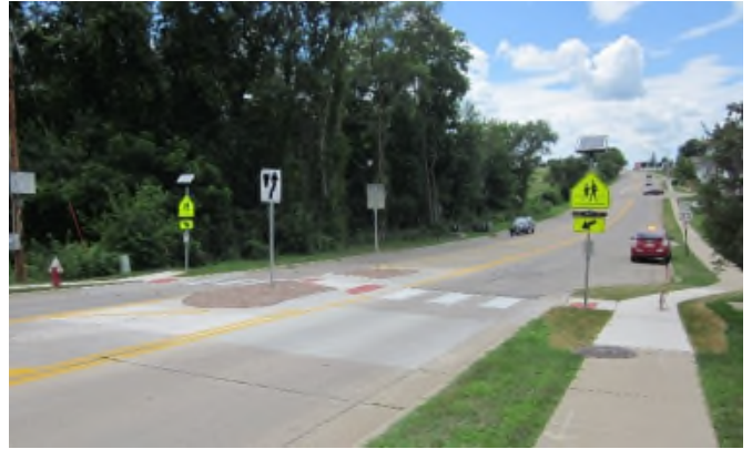
New Enhanced Sidewalk on Asbury Road
