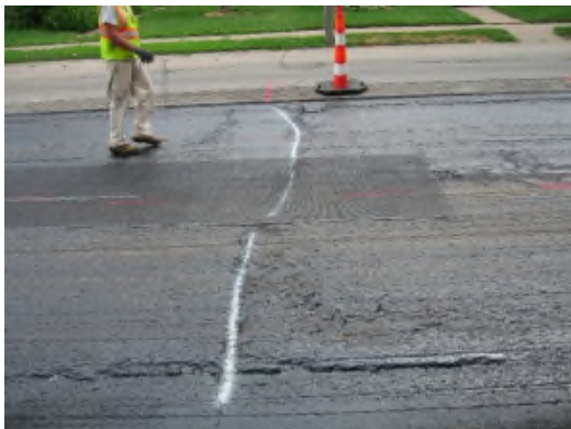
Installation of Geogrid over joints
