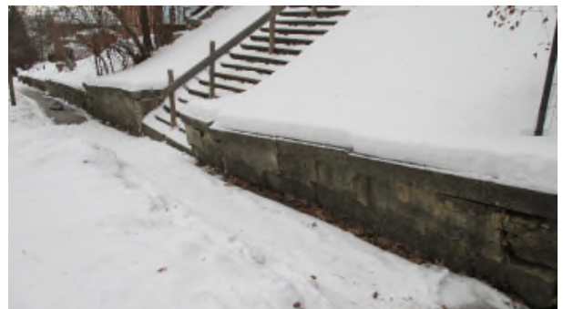
Sidewalk not shoveled
