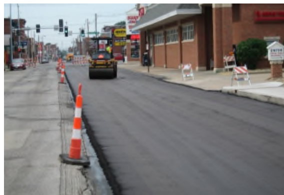
New Asphalt Interlayer Installed. Reduces Cracking.
